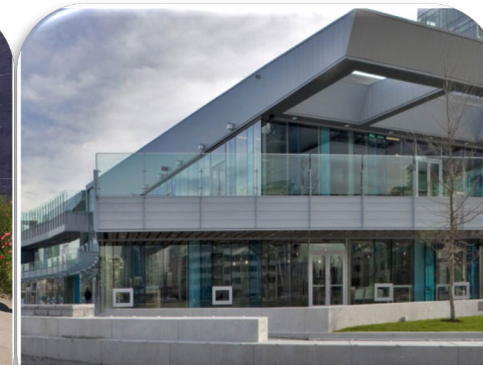
Creekside Community Centre
