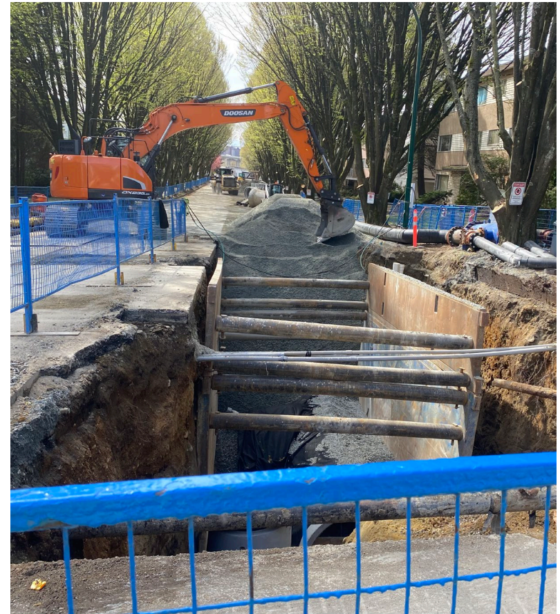
Oak St Sewer Separation Upgrade
