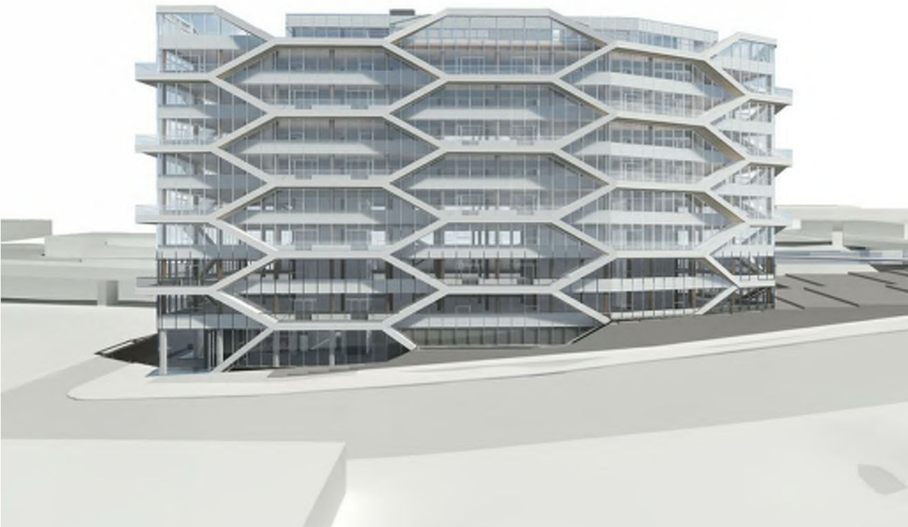
3. Balconies accentuate the braced frame structure as in the 2102 Keith Drive building
