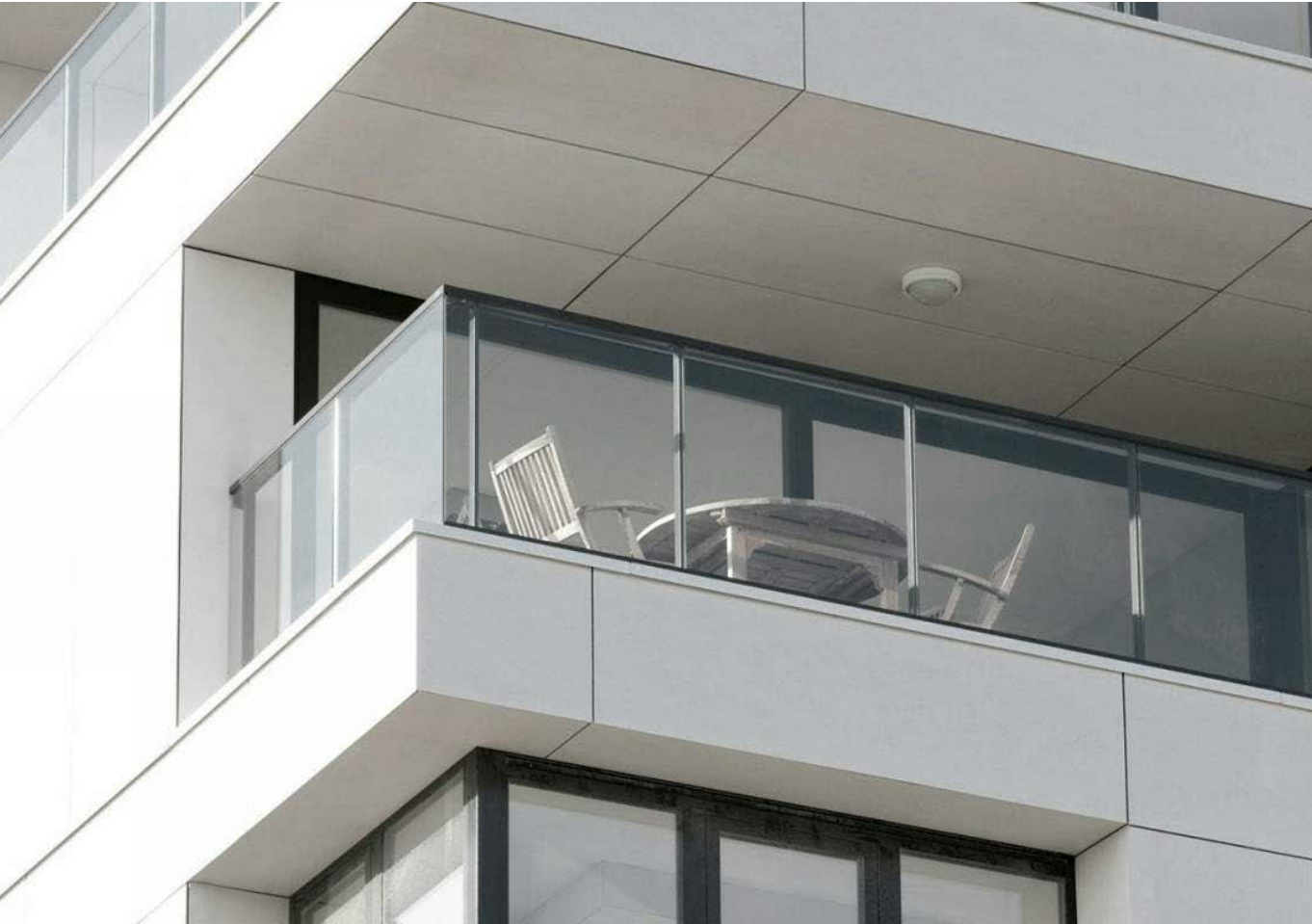
WHITE FIBRE CEMENT PANELS (2' X 10' PANELS)
