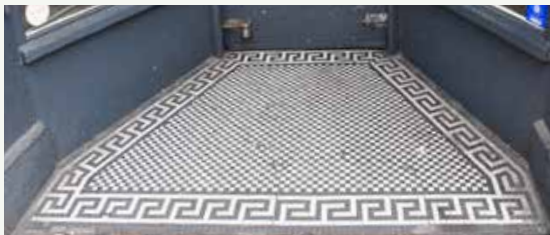
Black and white mosaic tilework in the recessed entryway on the chamfered corner. Luxton
