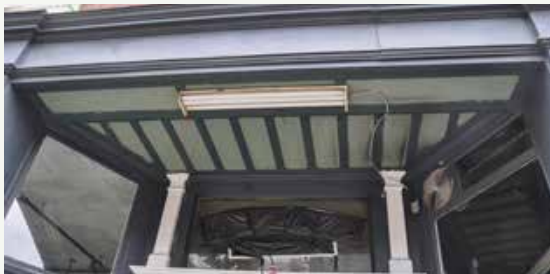
Wood soffit with recessed panelling in the recessed, primary entryway along West Pender Street. Luxton
