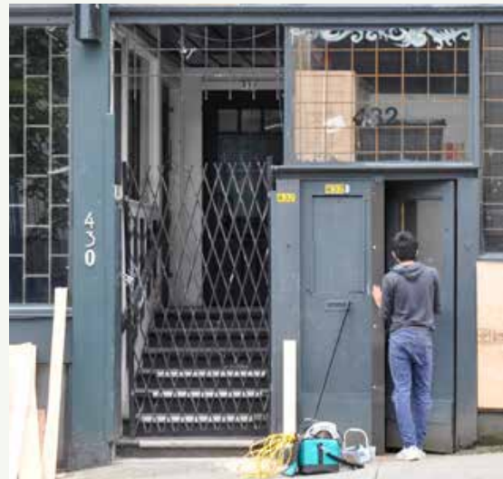
Wood storefront door (left) in recessed entryway, and later-addition double-doors with access to basement (right) along the Homer Street façade. Luxton
