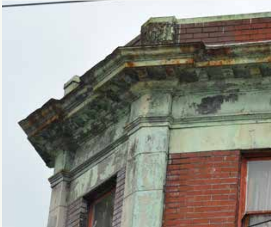
Sheet metal cornice along the chamfered corner of Hartney Chambers. Luxton
