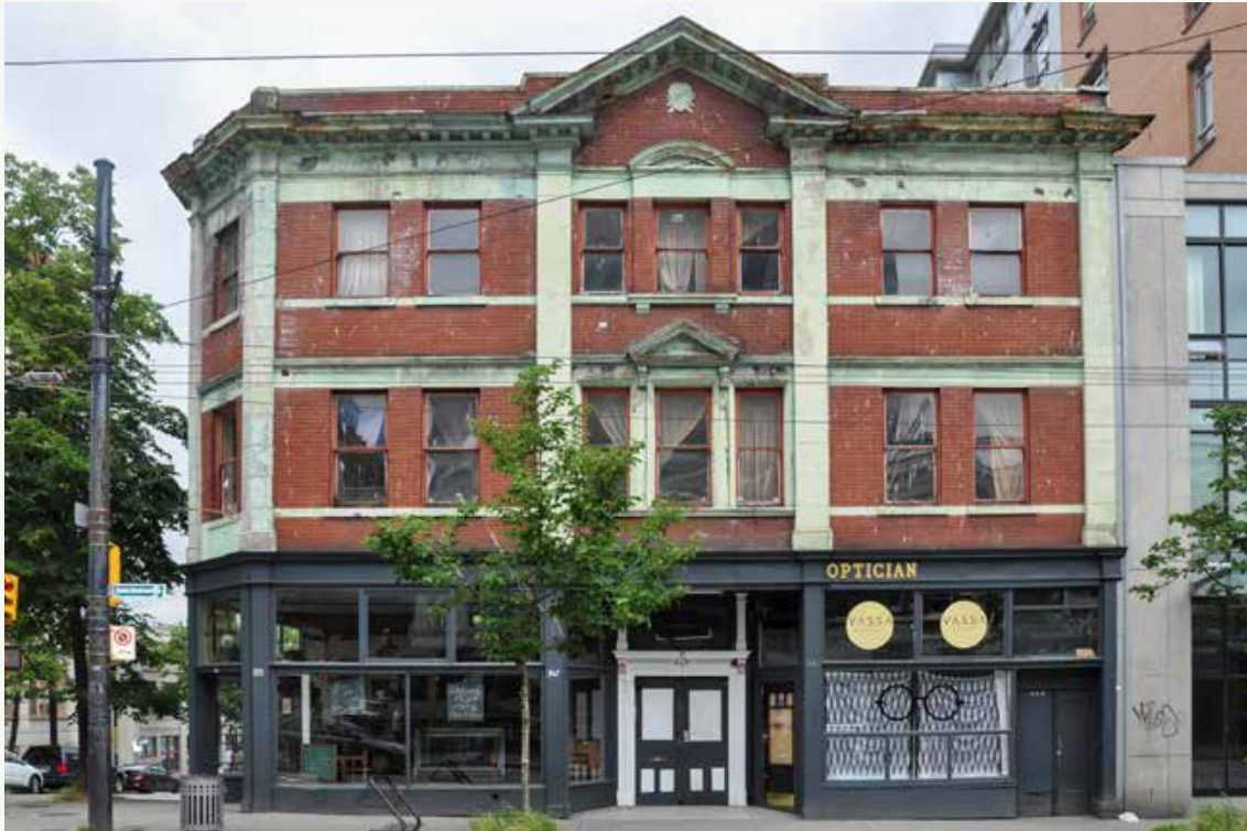
Architectural metal of the West Pender Street façade at the storefront cornice, window hoods, parapet cornice, and pediment of Hartney Chambers. Luxton
