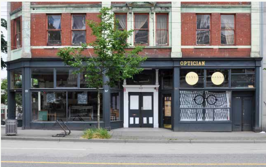
Storefront along West Pender Street with large plate glass storefront window, single-lite fixed and operable transoms. Some storefront glazing has been altered (far right) and the windows of the storefront bulkheads have been removed and/or covered over.
