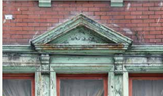
Sheet metal window hood above second storey window on West Pender Street façade. Luxton
