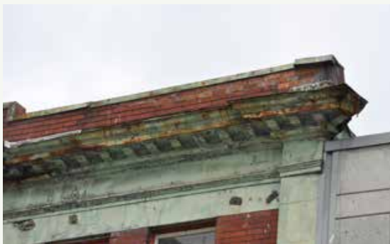
Deterioration of sheet metal rooftop cornice at southeast corner of Hartney Chambers. Luxton
