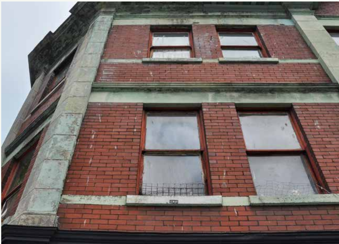
Oamaru stone pilasters, sills, and lintels of the West Pender Street façade of Hartney Chambers. Luxton
