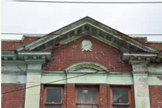
Large sheet metal open pediment on the West Pender Street façade. Luxton
