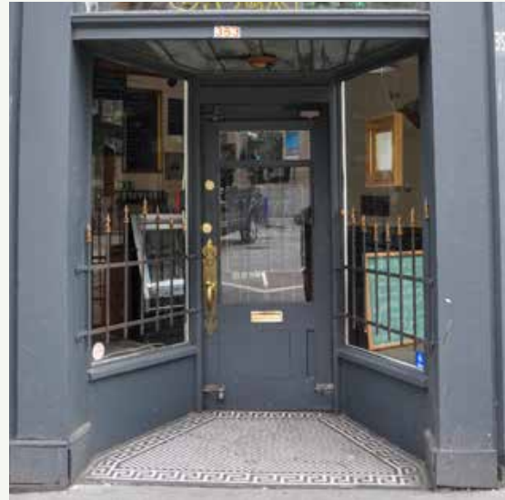
Wood door with glazing in the chamfered corner entry. Luxton
