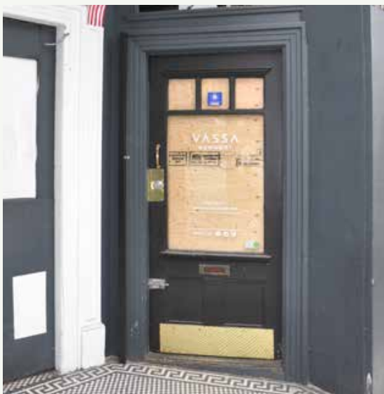
Wood storefront door in recessed entryway at West Pender Street. Luxton
