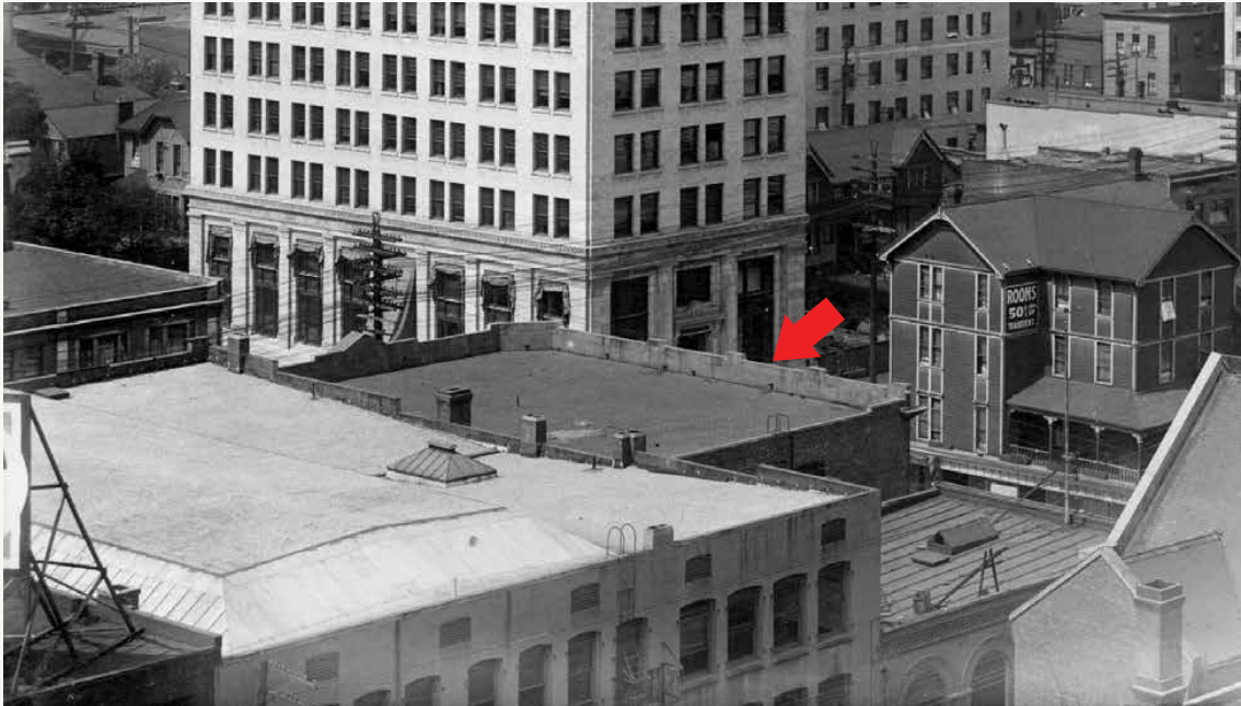
View of the roof of Hartney Chambers, note the narrowness of parapet with parged back, 1913. City of Vancouver Archives 371-727.1
