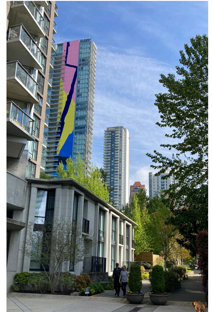
VIEW LOOKING NORTHEAST ON STRATHMORE MEWS
