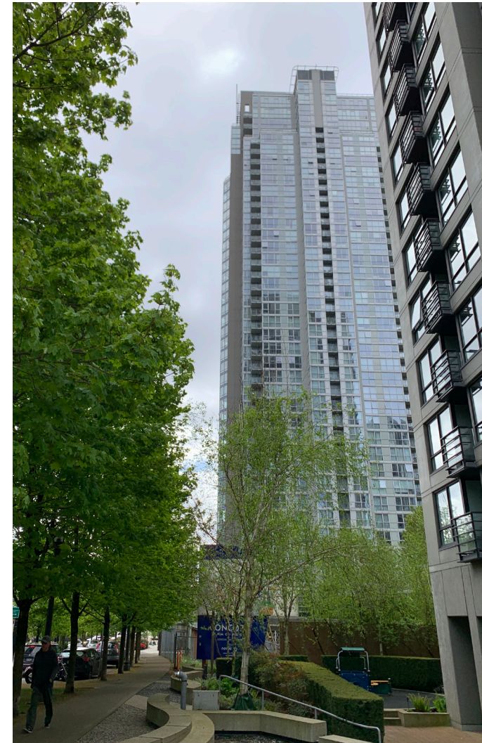
VIEW LOOKING SOUTHEAST ON PACIFIC STREET
