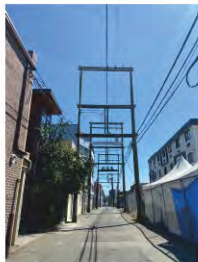
3 LANE - LOOKING EAST
