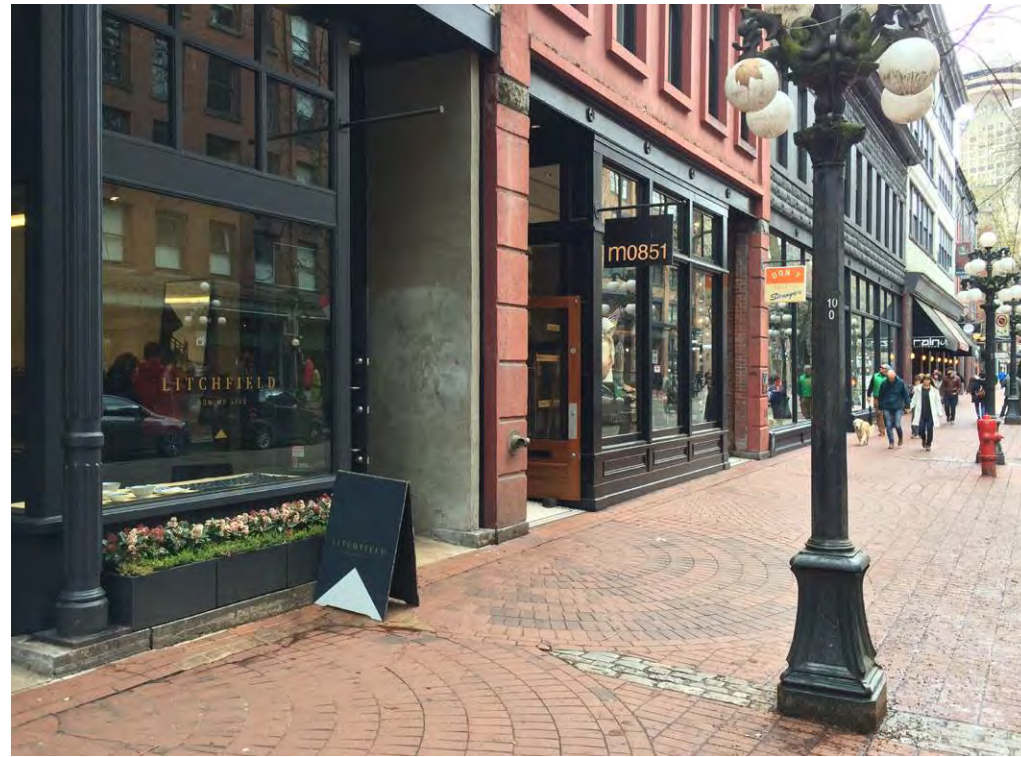
Gastown, Water Street: Continuous street front
