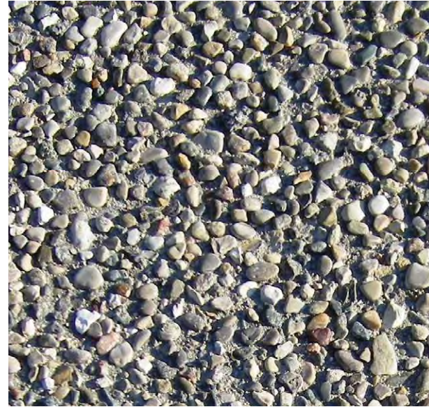
Exposed aggregate concrete Streetscape as per CoV standards
