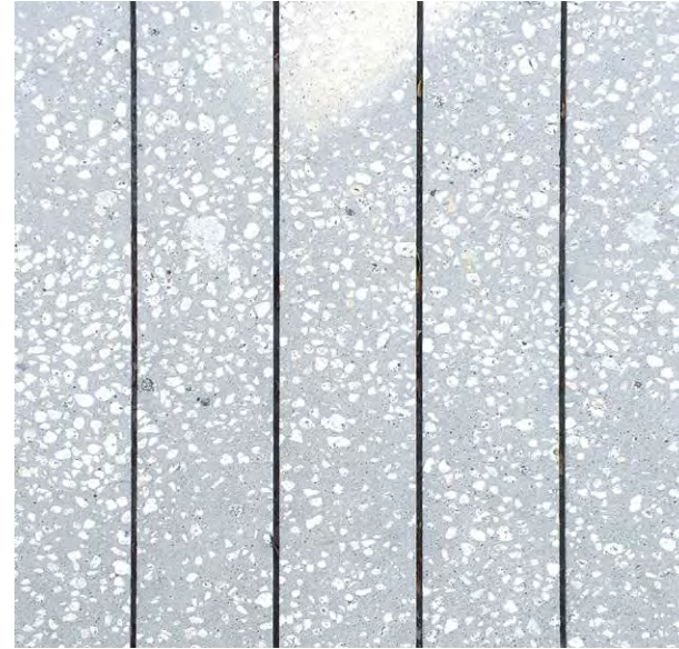
Precast concrete Planks Courtyard
