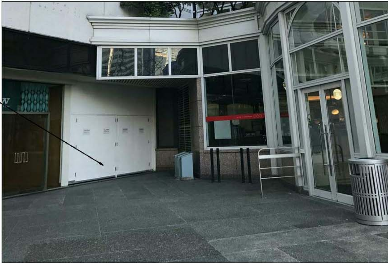
Existing hotel emergency exit doors and parkade exhaust
