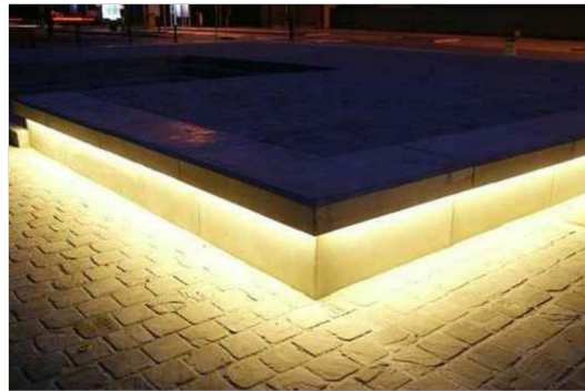
Light fixtures in overhang of planter wall direct light to the floor. The same detail could be used for the pool parapets.
