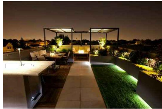
Light fixtures in overhang of planter wall direct light to the floor. The same detail could be used for the pool parapets.
