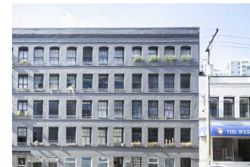
GRID OF WINDOWS IN NEIGHBOURING BUILDING (863-849 BEATTY STREET)
