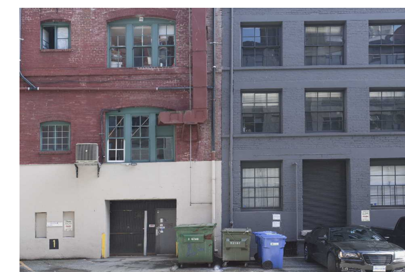
REAR LANE EXISTING CONDITION
