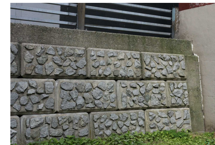
LOCK ROCK RETAINING WALL SEPARATING (LOWER) REAR LANE FROM (UPPER) SIDE LANE
