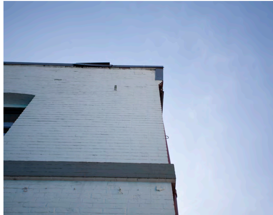
Existing roof cornice covered by metal flashing
