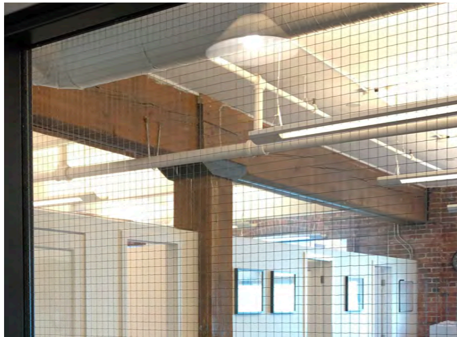
Existing heavy timber construction at 837 Beatty Street
