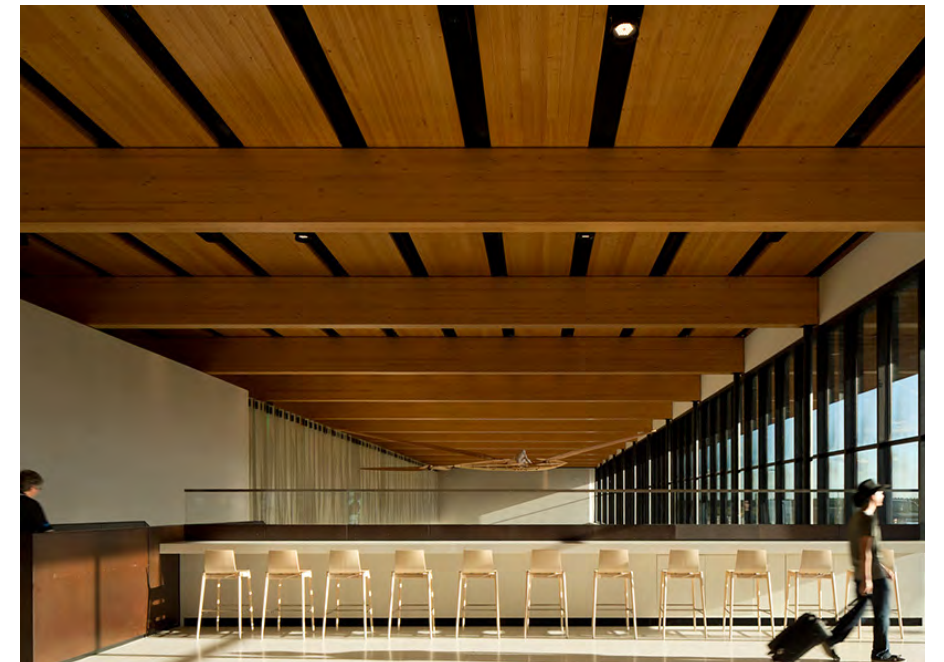
Examples of modern mass timber construction
