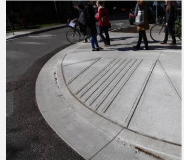
Grooves on broad apron curb cuts
