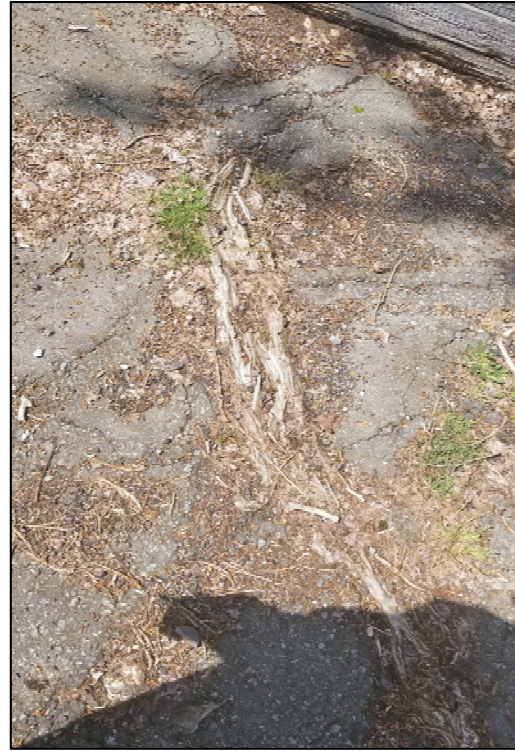
Image 5 - Structural roots extending through asphalt
