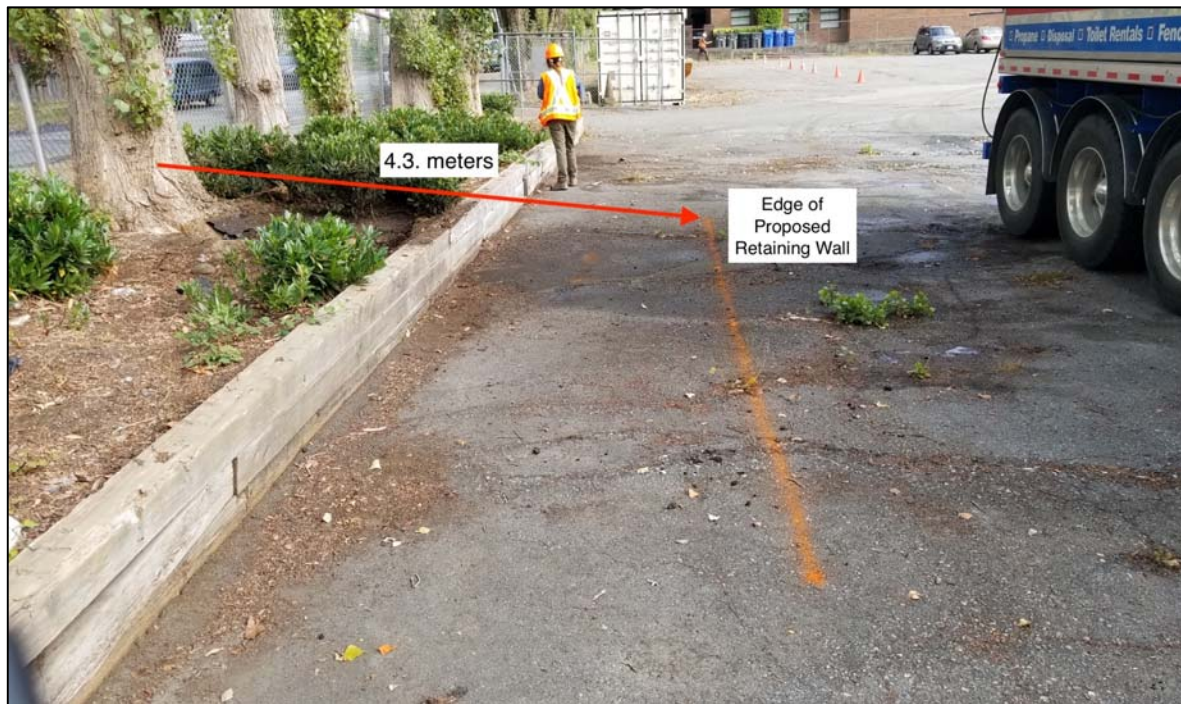
Fig. 1 – View of edge of proposed retaining wall, which is located 4.3 meters from the edge of poplars' trunks
