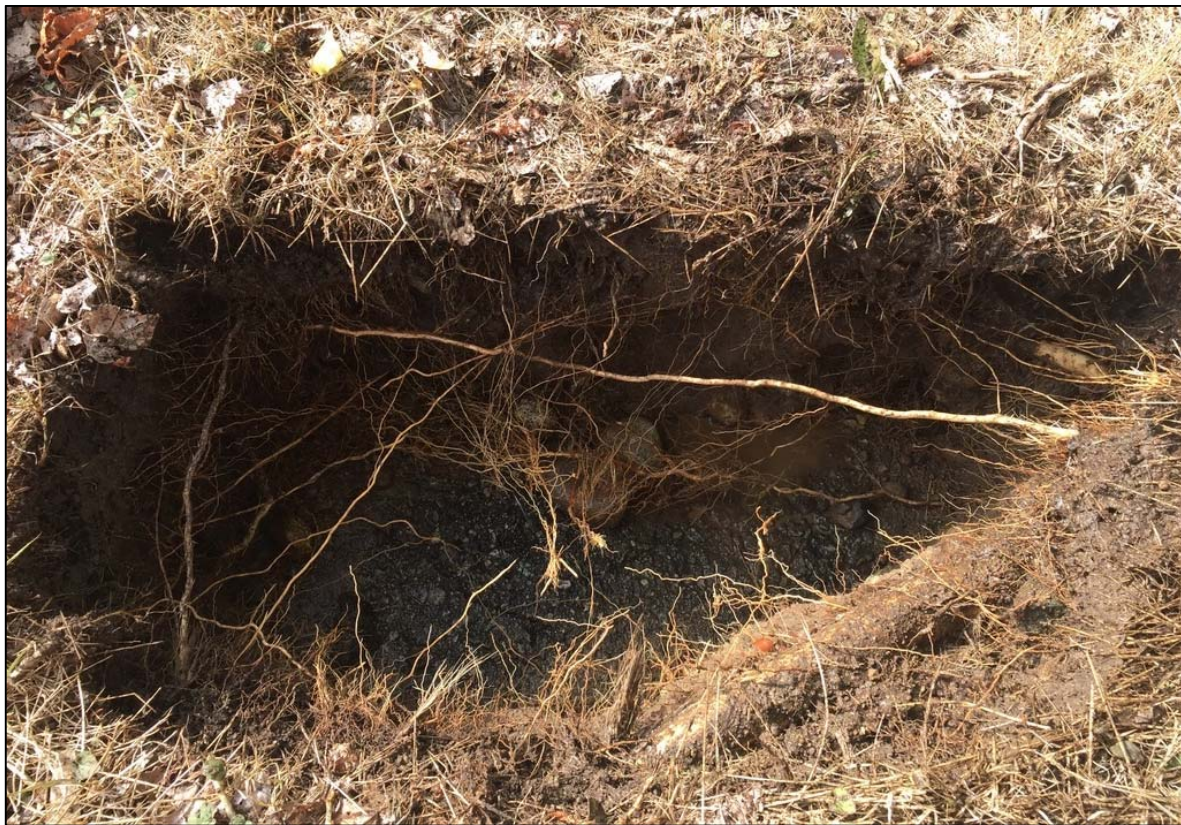
Fig. 2 – Excavated trench east of Tree 034, which uncovered a layer of asphalt 0.5 meters from the surface
