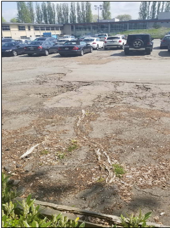
Image 4 - Cracks and lifting of asphalt.
