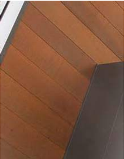
Cedar soffits at canopy over sidewalk
