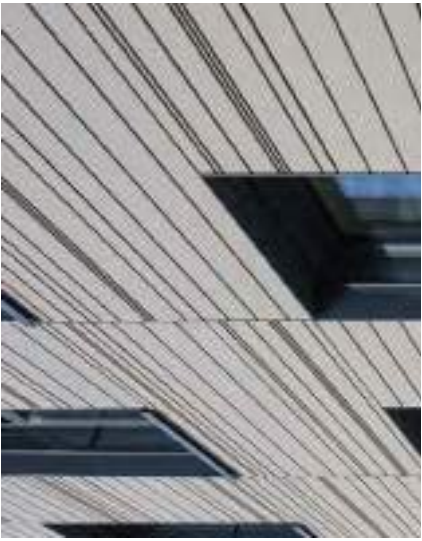
Longhouse - Cladding in cementitious or terracotta plank panels
