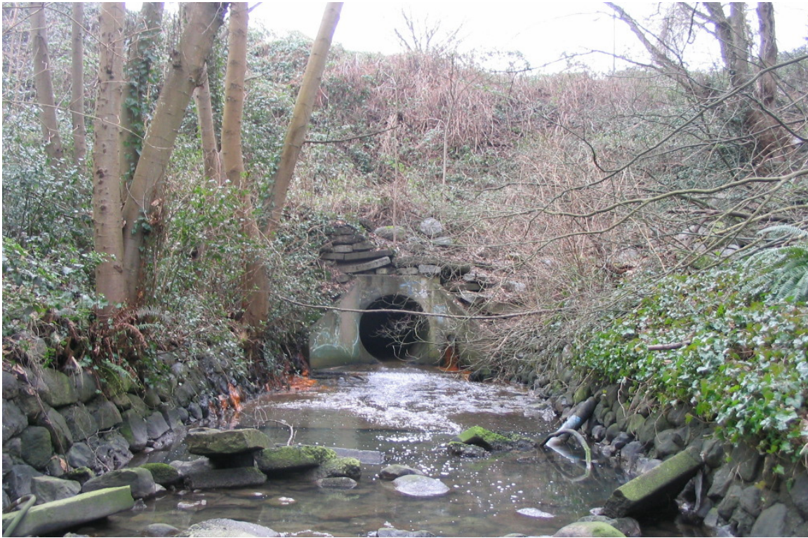
Photo 1 Looking upstream at 29 th Avenue stormsewer outlet
