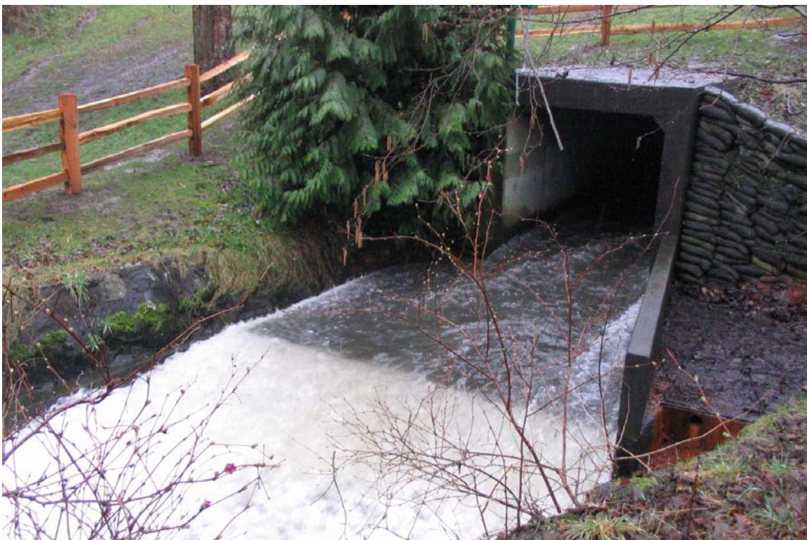
Photo 10 Outlet of 22 nd Avenue culvert under higher flows
