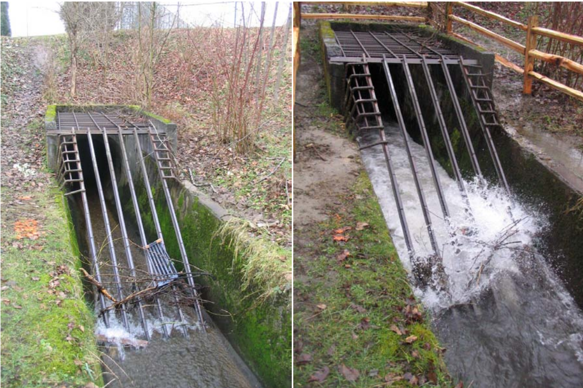
Photo 16/17 Looking downstream at debris rack under low flow on the left and higher flow on the right. Note the debris on the rack.
