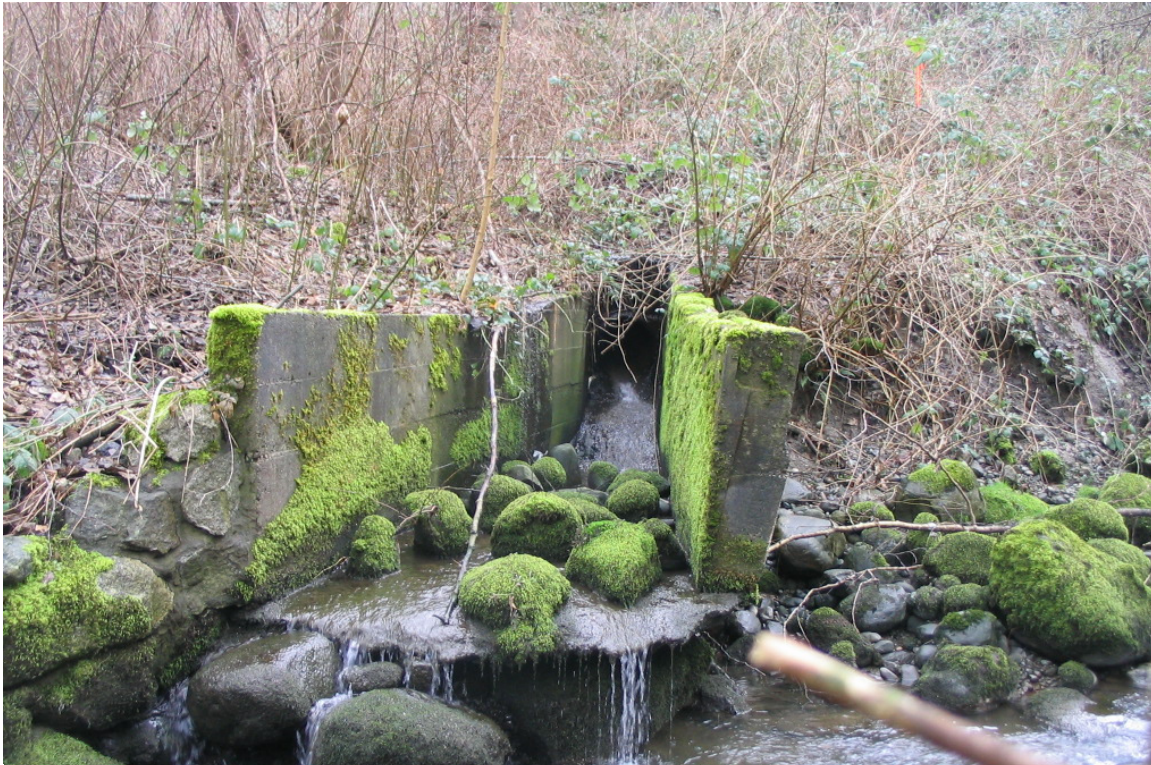
Photo 5 Looking at stormwater outfall at 26 th Avenue – note the channel incision since construction
