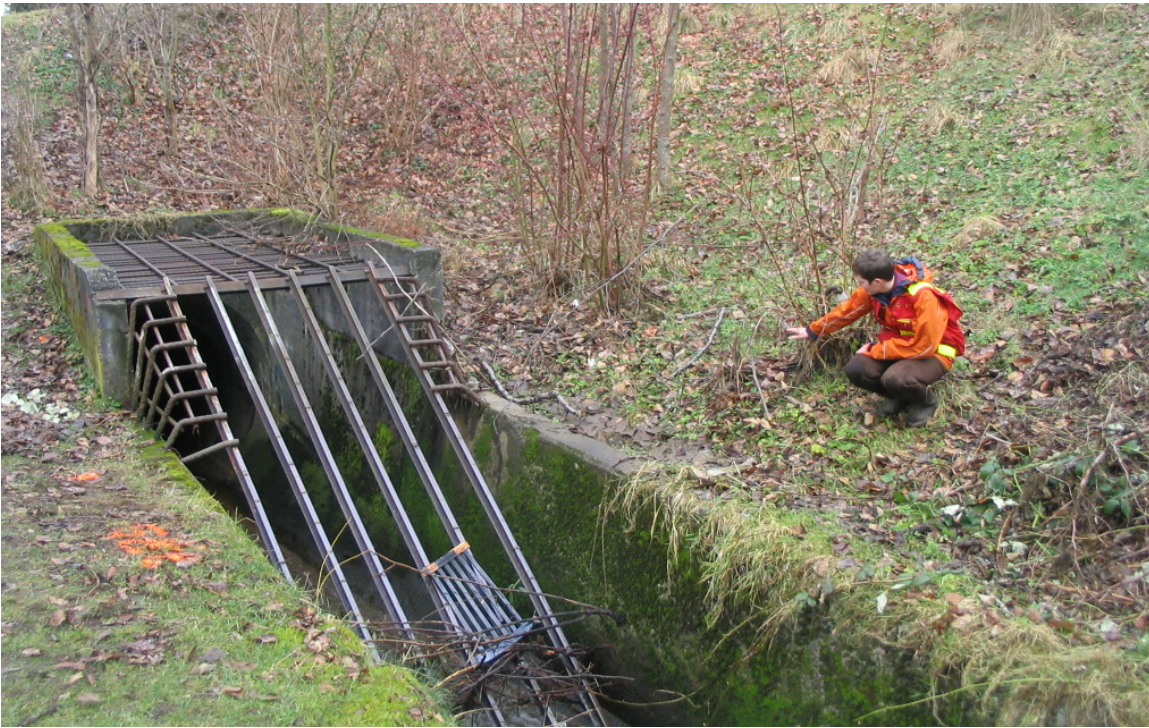
Photo 15 Renfrew Street culvert inlet – note rafted debris indicated in the field near the top of debris rack
