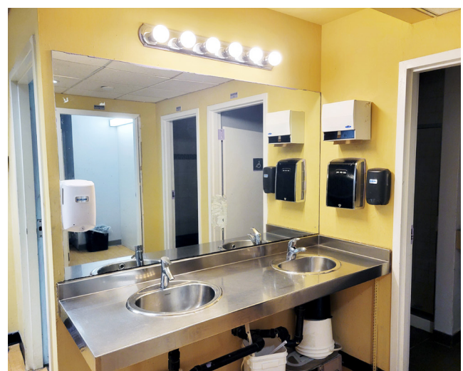
Bathroom renovation at Downtown Eastside Women's Centre
