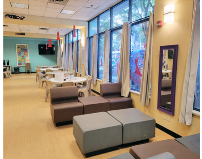
Renovation at the Drop-in Centre/ Downtown Eastside Women's Centre
