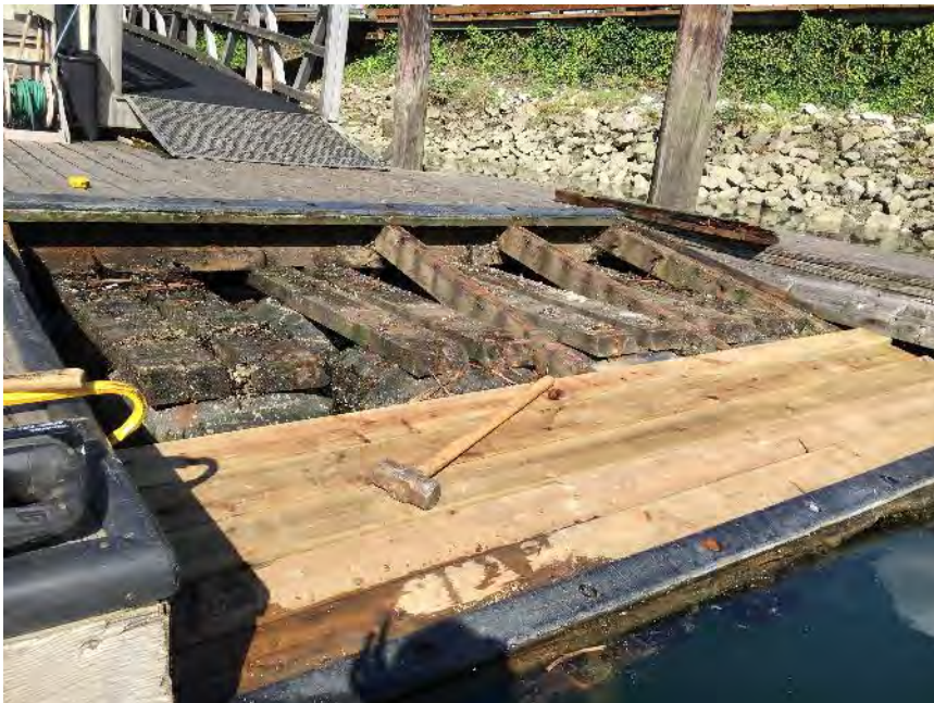
Photo 8 Exposed structural timber at northeast end of timber float.
