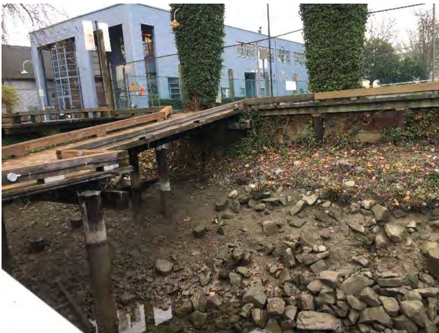
Photo 4 Minor weathering deterioration to timber pile caps and piles.
