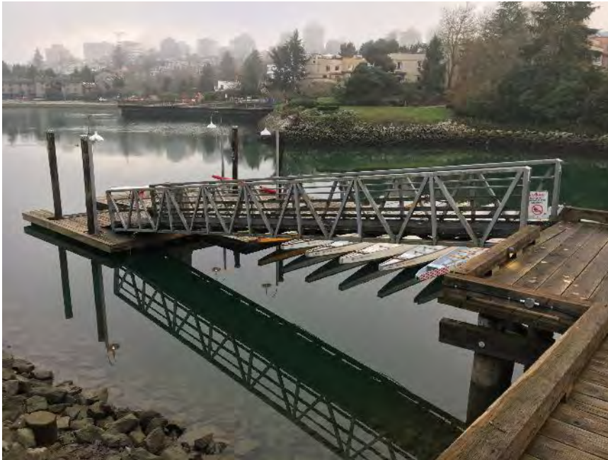
Photo 5 Aluminum gangway in a serviceable condition.
