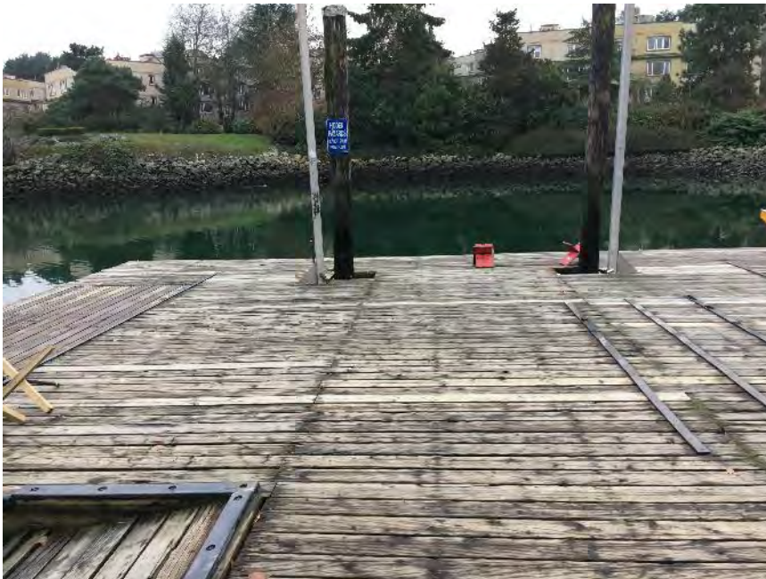
Photo 6 Moderate weathering deterioration to deck planks on float.
