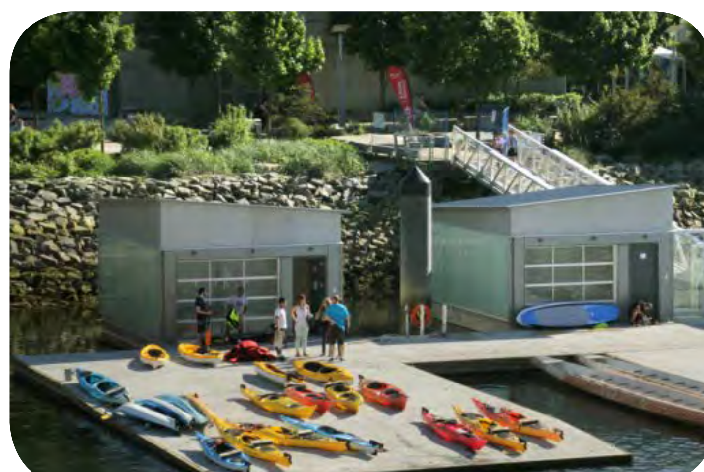
Tapered concrete dock / float
