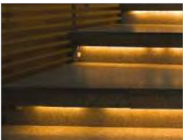
LED STRIP LIGHT UNDER THE STEPS
