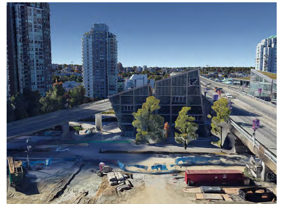
Site View Towards South (Google Earth)
