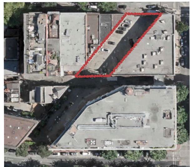
Aerial view of the site showing the existing condition
