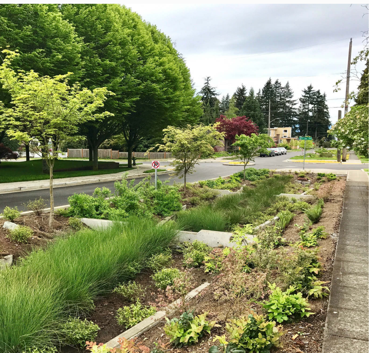
Bioswale Venema Creek, Seattle Reconstructed 5 city blocks to collect and manage stormwater from more than 80 acres.
