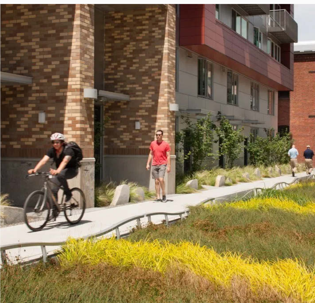
Bioswale Yale Street, Seattle Treats 190 million gallons of stormwater annually
