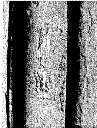
Closeup view of peeling paint of the east wall
