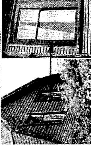
Replacement windows of the east façade – new, wood sash windows should be fabricated to match the double-hung wood sash windows with decorative horns found elsewhere on the building, identical to the photo on the right
