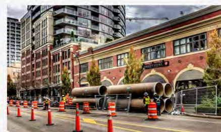
Columbia Street mainline sewer separation in progress. (Photo credit: Dennis Sylvester Hurd via flickr , CC BY 2.0)
