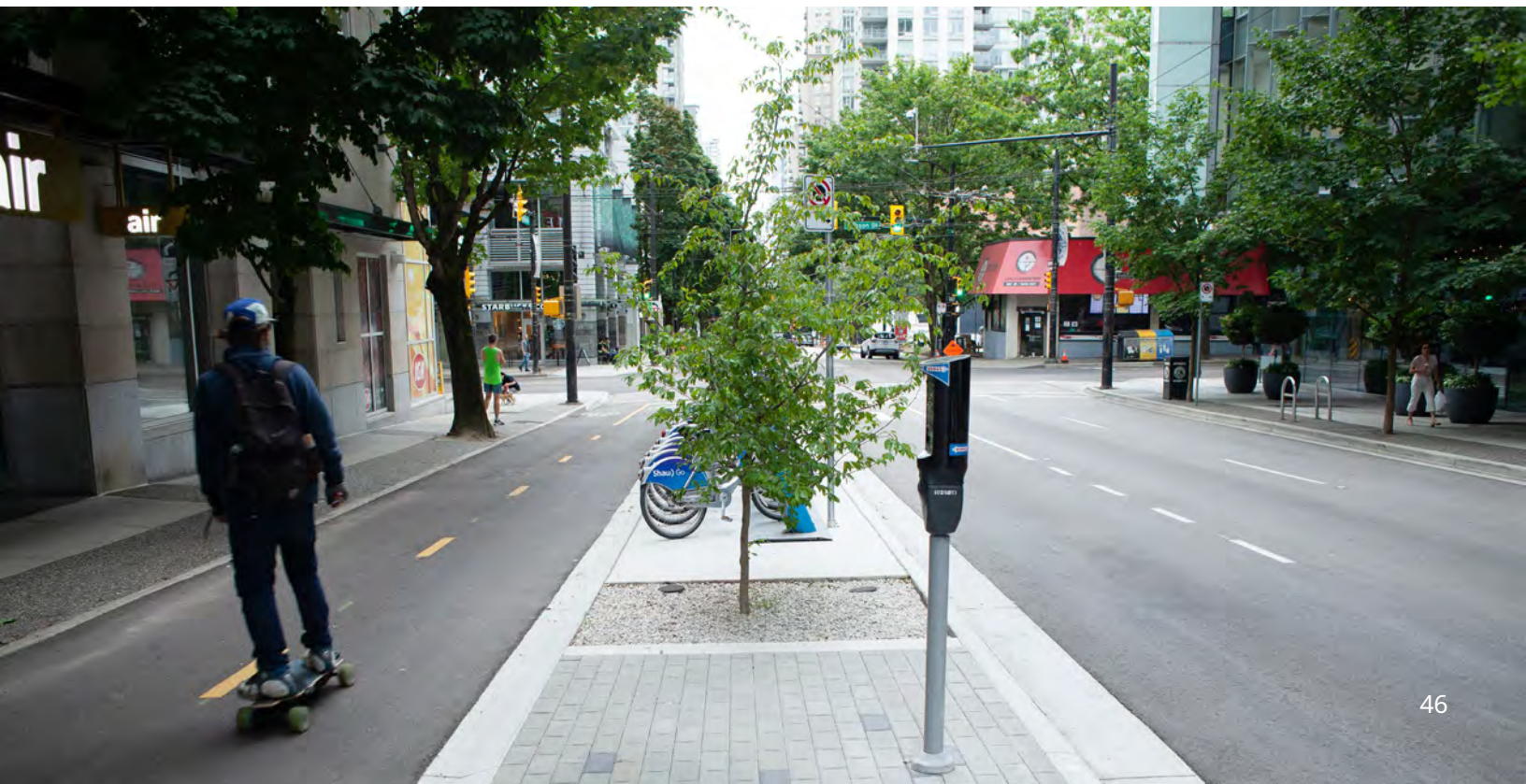
Figure 20: Bioretention bulge (a Green Street feature) at 14 th and Woodland, Vancouver
