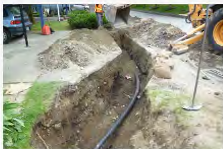
Separating a sewer lateral. (Photo credit: KWL)
