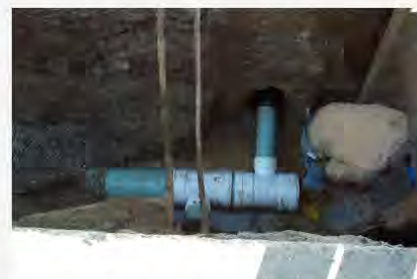
Sanitary sewer replacement and separating/replacing a combined private sewer lateral (Photo Credit: Pam Broviak) 2
