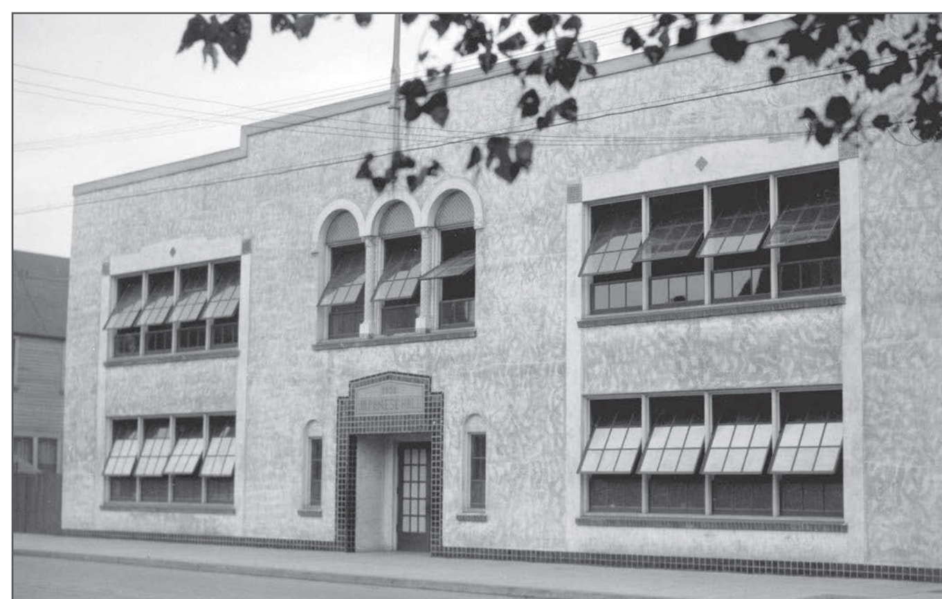
Japanese Hall at 475 Alexander Street (1929) Vancouver Archives AM1535 99-2469
