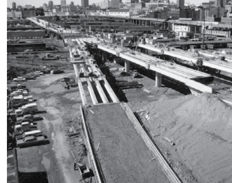
Construction of Georgia Viaduct in 1970
