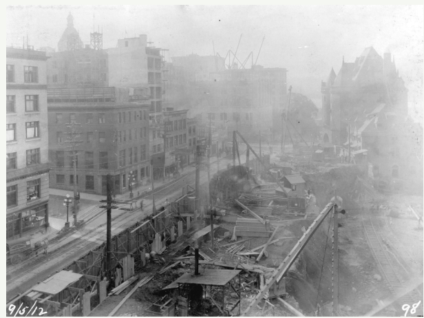
1912 construction views of the CPR Station, showing the excavation and staged erection of the steel structure. (CVA 152-5 series)
