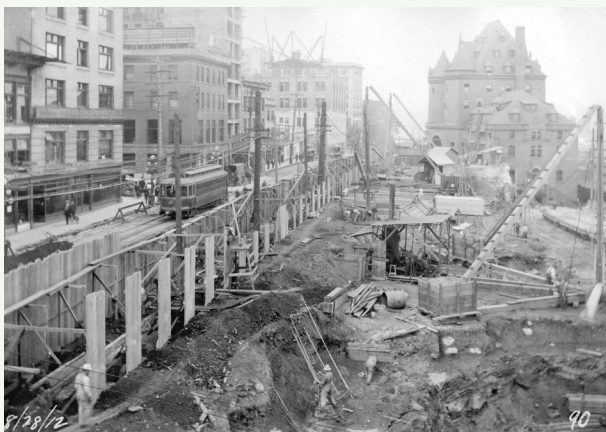
1912 construction views of the CPR Station, showing the excavation and staged erection of the steel structure. (CVA 152-5 series)
