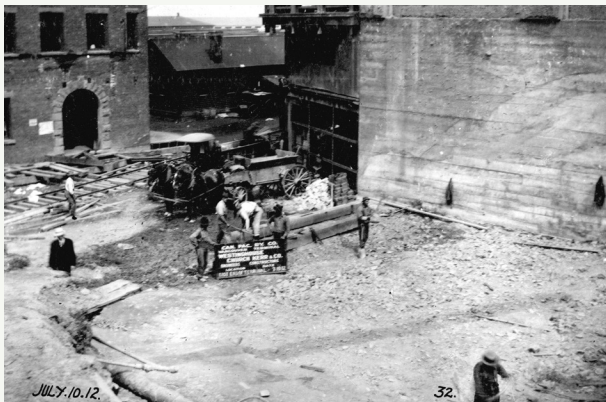
1912 construction views of the CPR Station, showing the excavation and staged erection of the steel structure. (CVA 152-5 series)
