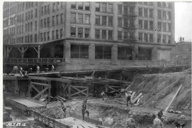
1912 construction views of the CPR Station, showing the excavation and staged erection of the steel structure. (CVA 152-5 series)
