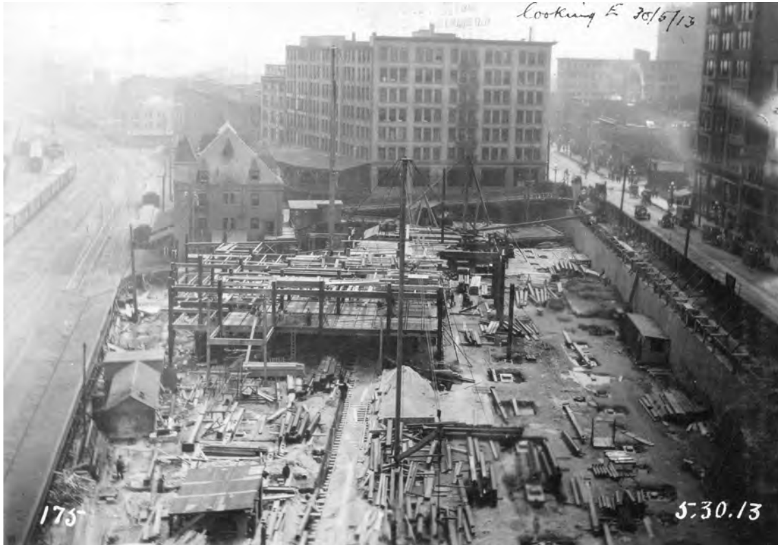
1913-05-30. CPR Station under-construction [CVA 152-1.155]
