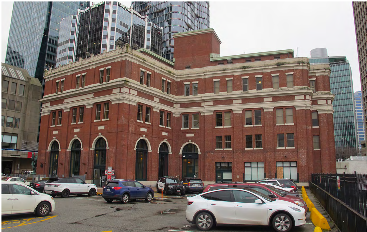
East elevation of CPR Waterfront Station
