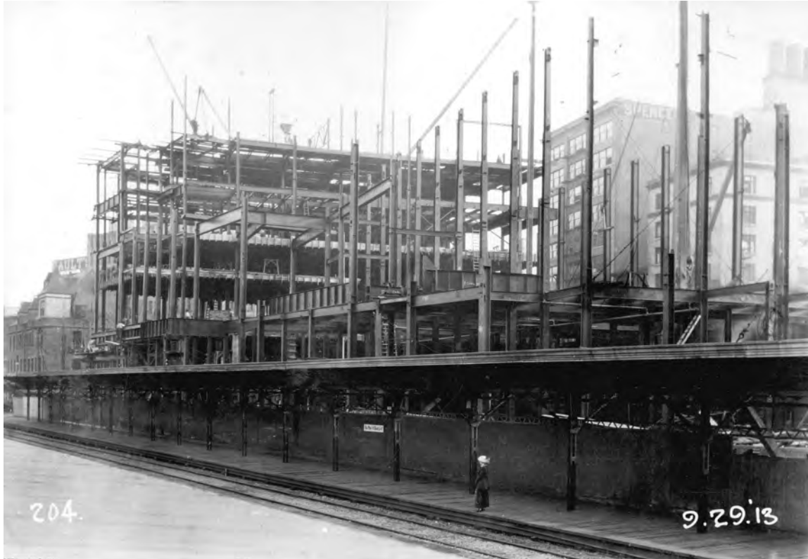
1913-09-29. CPR Station under-construction [CVA 152-1.033]
