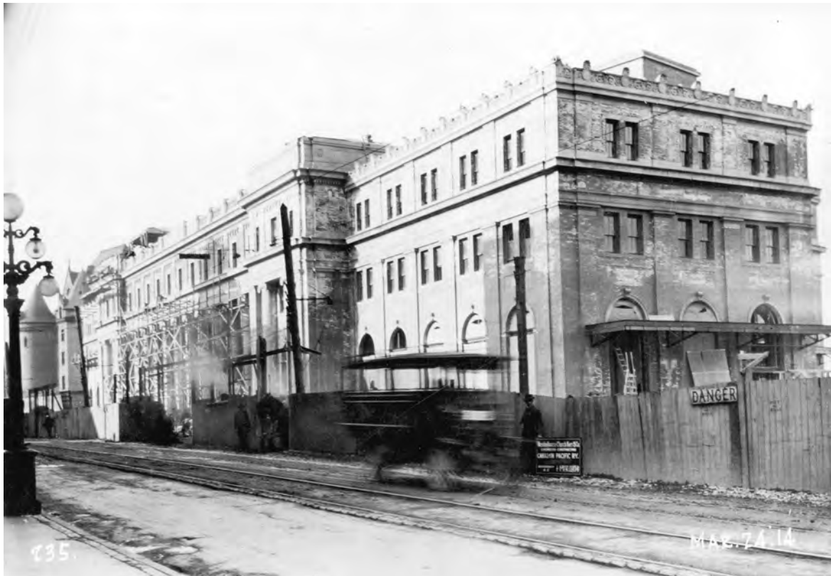
1914-03-24. CPR Station under-construction [CVA 152-1.063]
