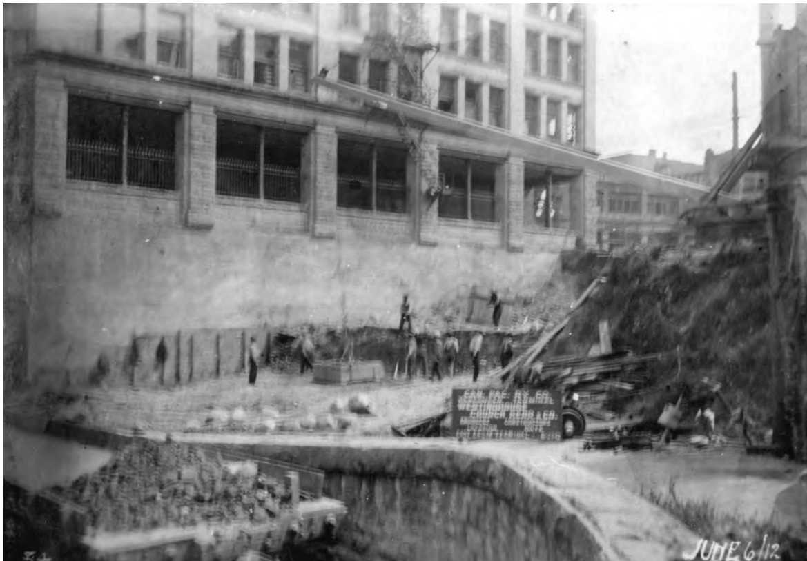
1912-06-06. CPR Station under-construction [CVA 152-5.022]
