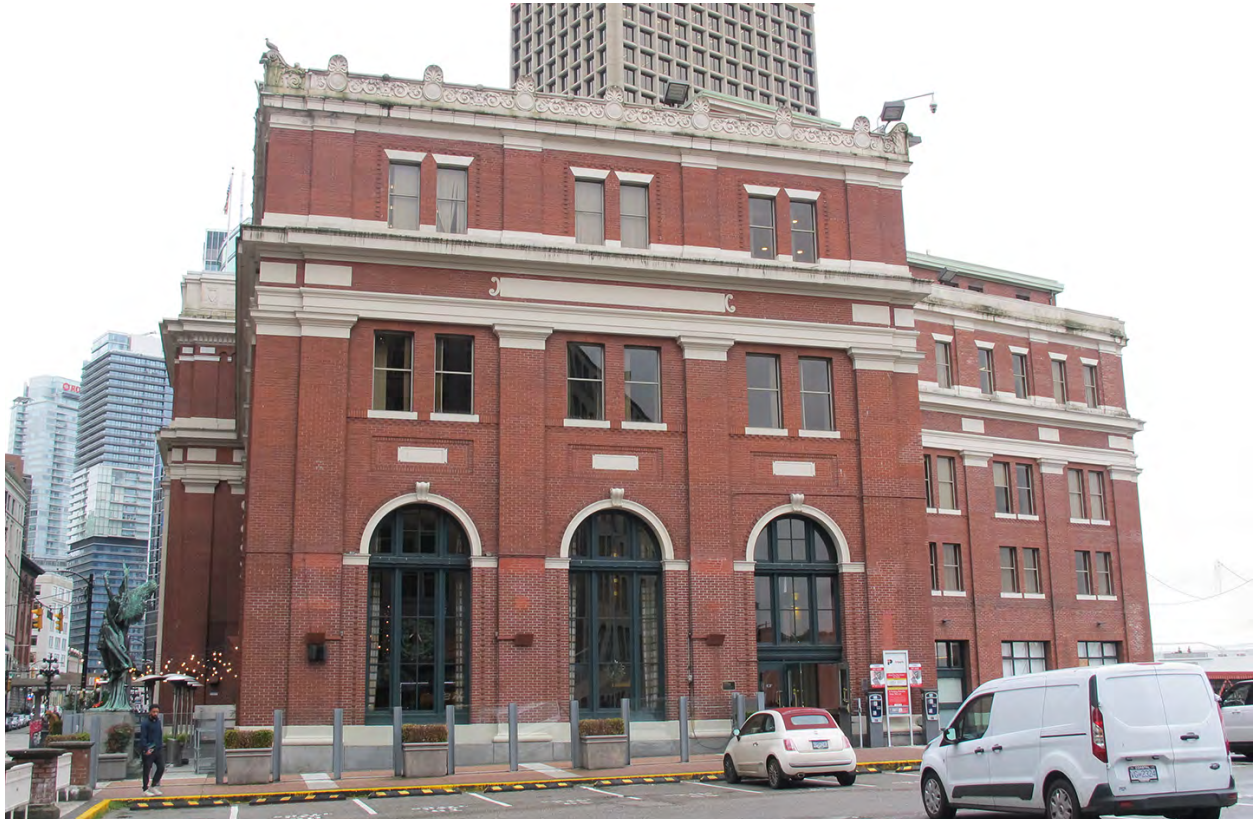
East elevation of CPR Waterfront Station
