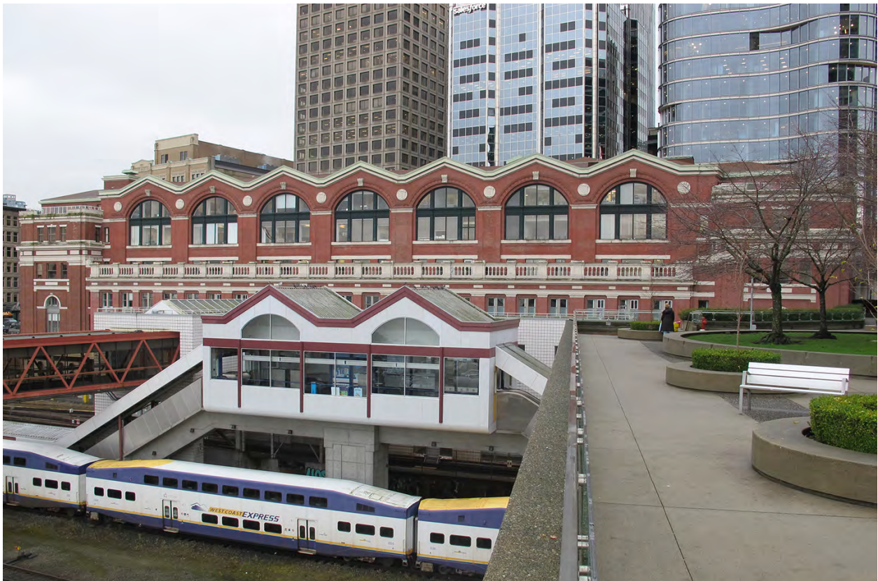
Rear elevation of CPR Waterfront Station from the Granville Square lookout
