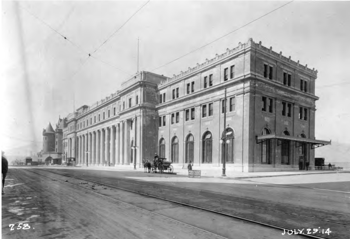
1914-07-29. CPR Station under-construction [CVA 152-1.080]
