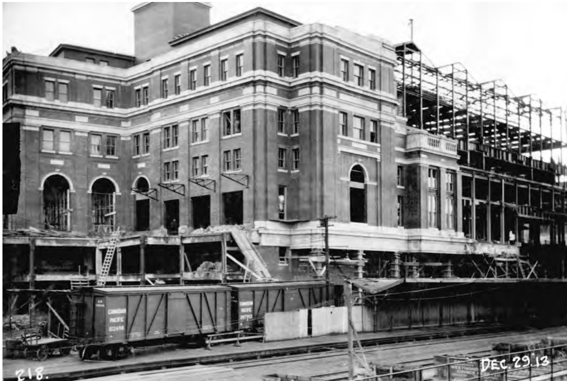
1913-12-29. CPR Station under-construction [CVA 152-1.055]
