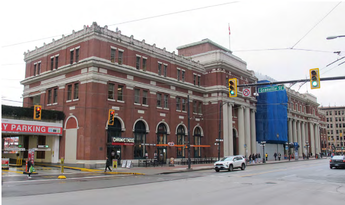
Front elevation of CPR Waterfront Station
