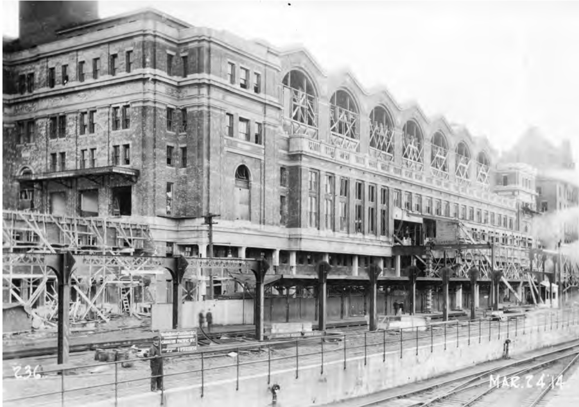
1914-03-24. CPR Station under-construction [CVA 152-1.064]
