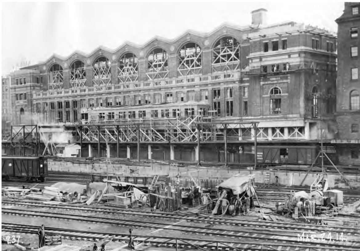
1914-03-24. CPR Station under-construction [CVA 152-1.209]
