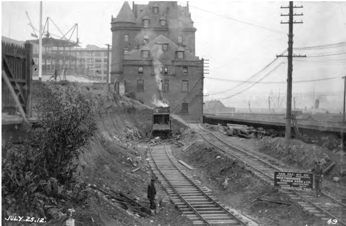
1912-07-25. CPR Station under-construction [CVA 152-5.031]
