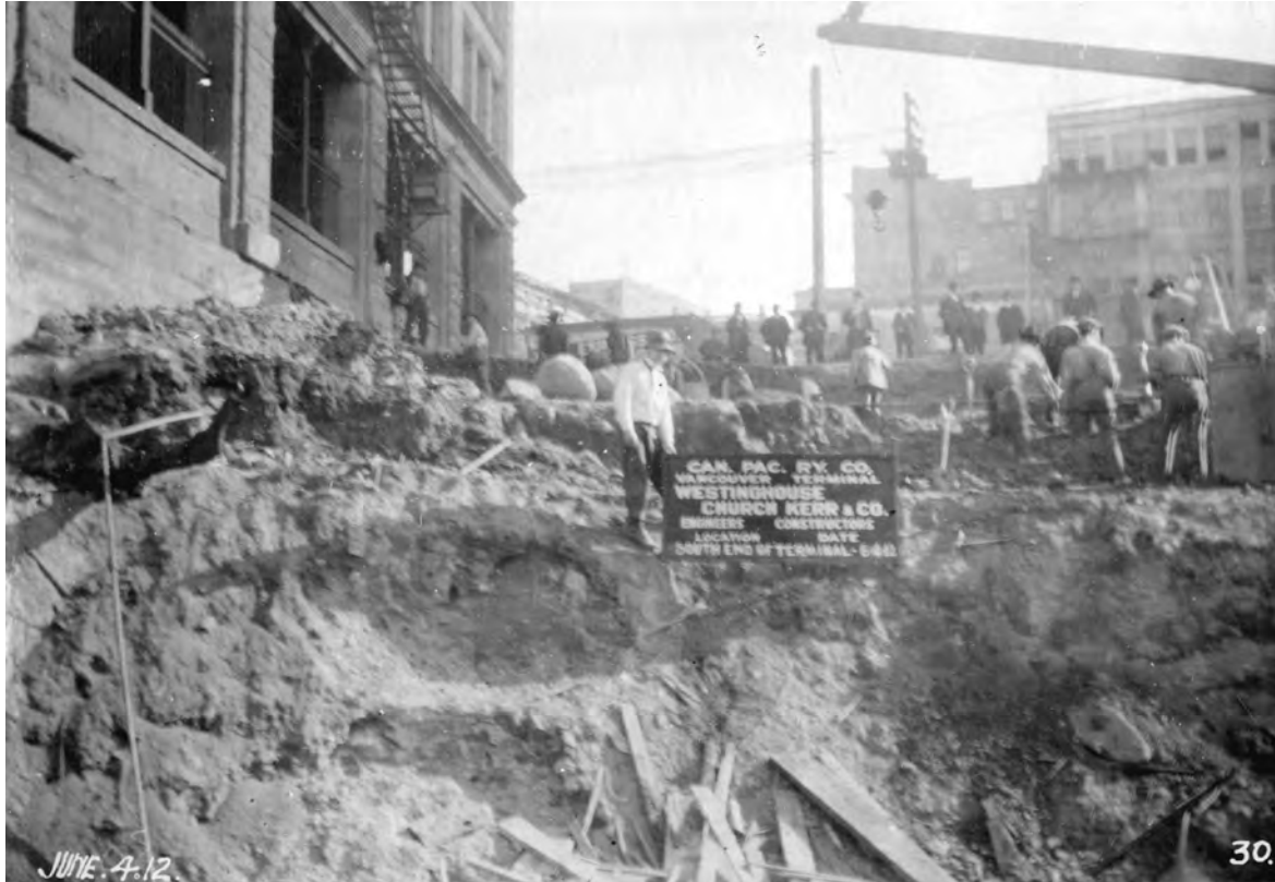
1912-06-04. CPR Station under-construction [CVA 152-5.021]
