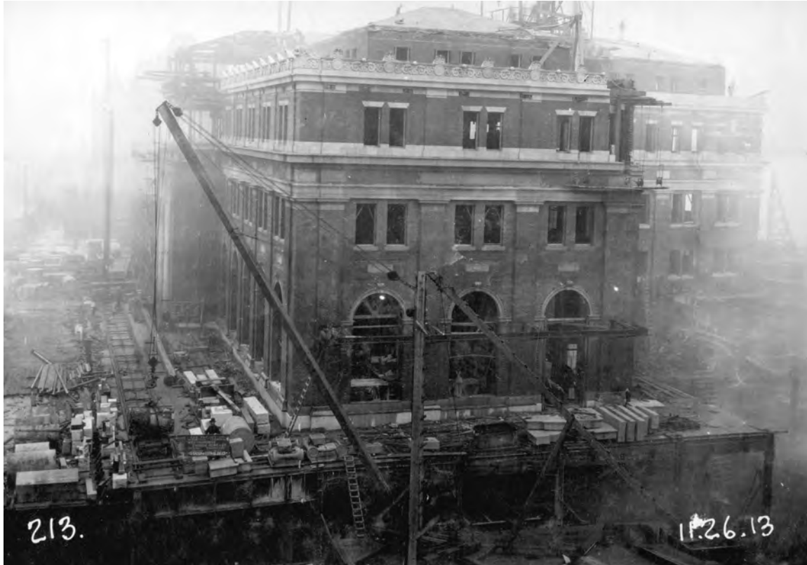
1913-11-26. CPR Station under-construction [CVA 152-1.052]
