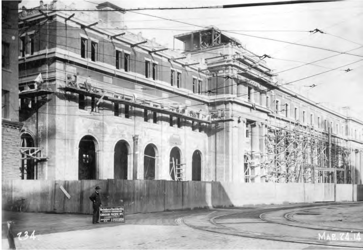
1914-03-24. CPR Station under-construction [CVA 152-1.062]
