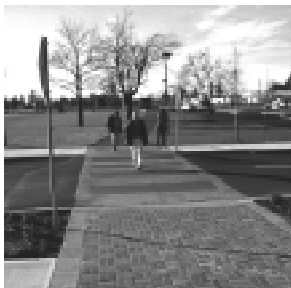
Speed table: raised pavement slows traffic (Portland, Oregon)
