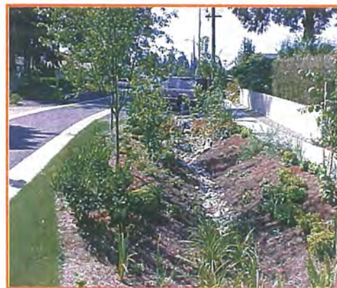
Managing Rainwater naturally – street side vegetated swales.
