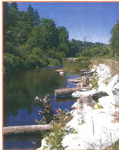
Bioengineering of stream bank
