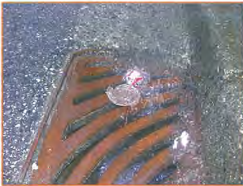
Streets are directly connected through pipes to watercourses
