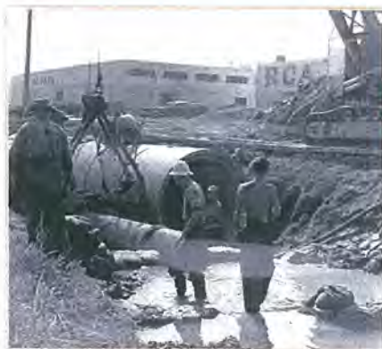
Placing the culvert to enclose Still Creek – Vancouver, 1955
