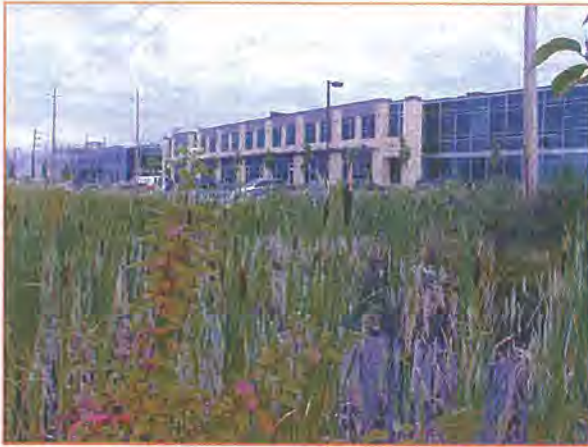
In Bridge Business Park, Burnaby, this constructed wetland filters water before it enters Chub Creek, a tributary to Still Creek. The wetland also provides aesthetic and habitat benefits for the area.
