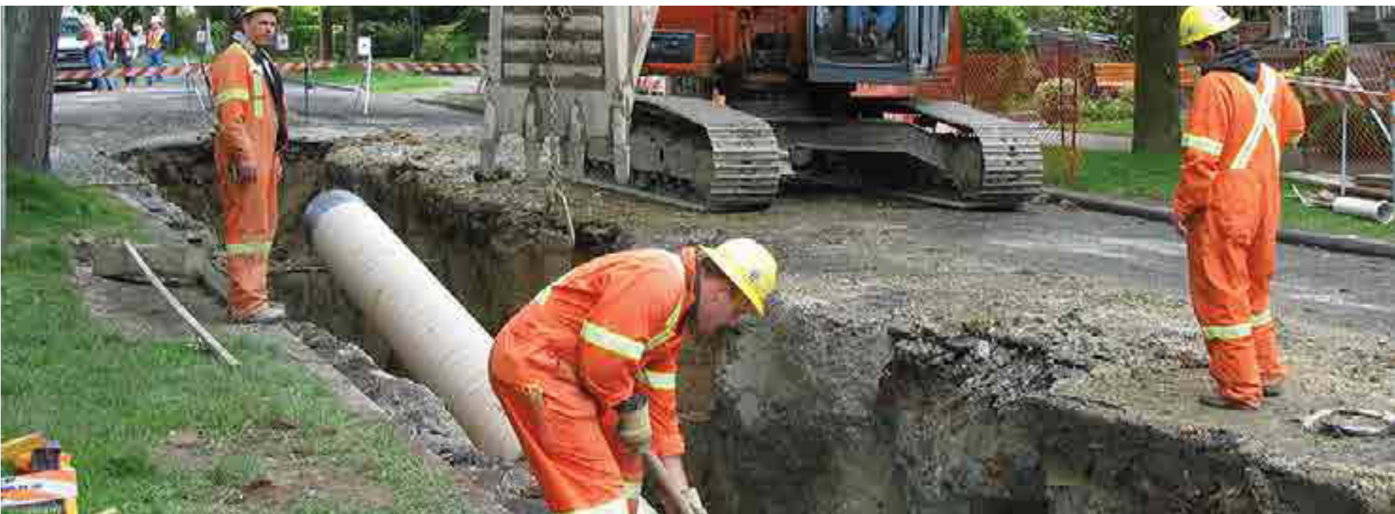
Separating sewage from rain water
