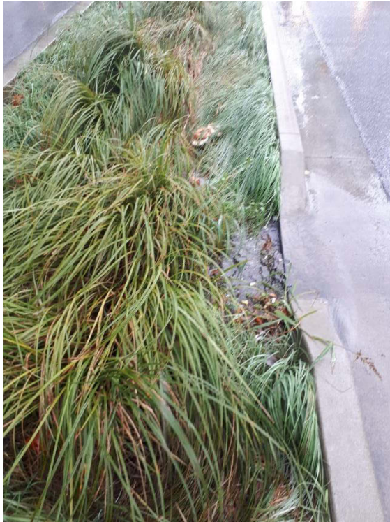
Photo of inlet ponding at Quebec & 1 st Location D during rain event
