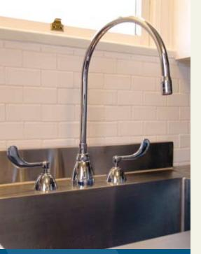
Reduce the risk of scalding–and save energy–by using antiscald devices. Also, install or upgrade insulation on hot water pipes. This will reduce heat loss from water heater to point of use.
