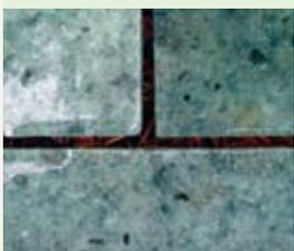
Recycled glass is re-melted into forms, creating hefty, translucent pavers; can be laid similar to concrete pavers, or interspersed as accent pieces with traditional stone or concrete products. Due to their recycled content, glass pavers require roughly half the energy necessary to create new, similarly performing concrete pavers.
