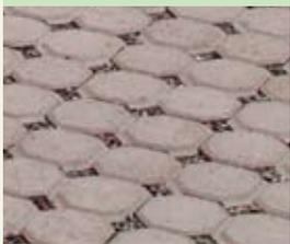
Concrete paving creates impervious surfaces that increase stormwater runoff. Look for interlocking concrete pavers in permeable designs that allow rain to seep between the pavers. Also consider installing conventional salvaged pavers to allow for rain infiltration.
