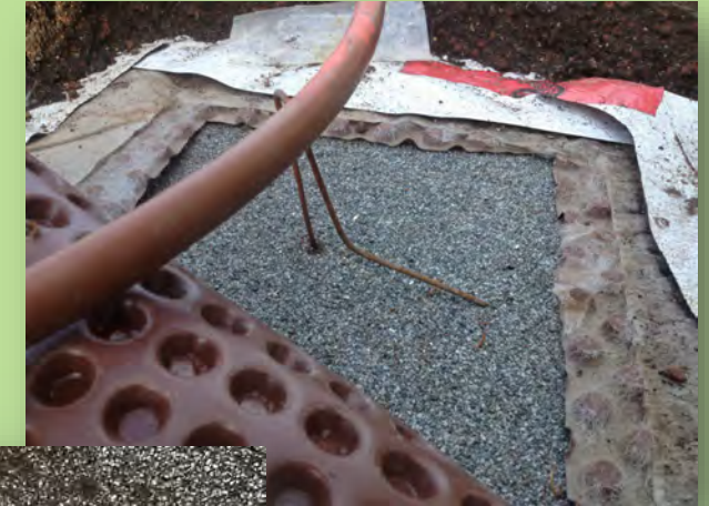
Irrigation support driven through roof waterproofing membrane Photo credit: RCABC
