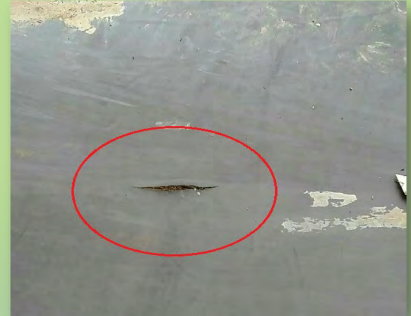
EPDM (“rubber”) roof membrane damaged by landscaper’s tool
