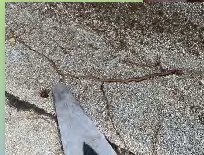
Root damage to membrane (six years, no maintenance) Photo credit: RCABC
