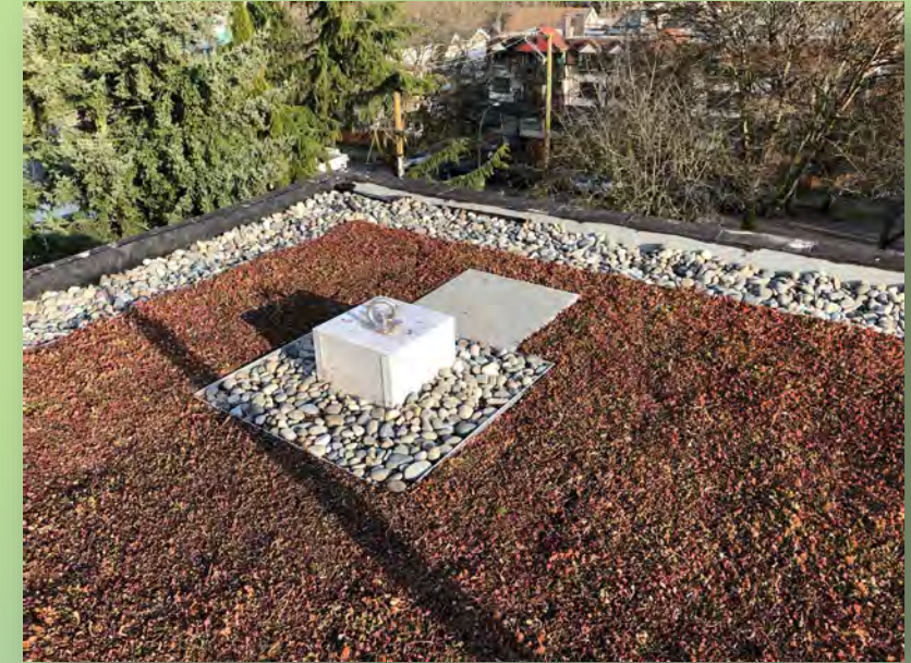
Example of separation zones around details and perimeters Photo credit: Architek Sustainable Building Products Inc.
