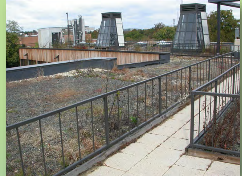
A dead green roof Photo credit: Unknown
