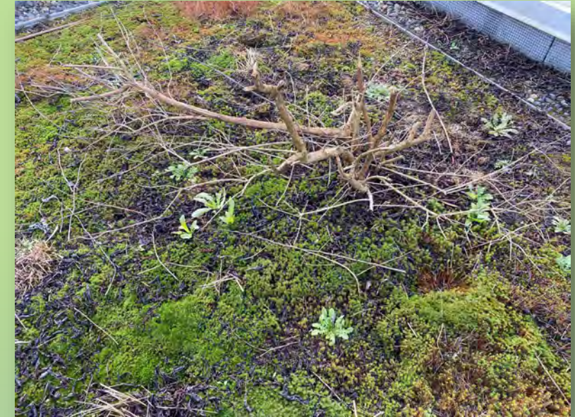
Burnaby sedum roof – left unmaintained for six years
