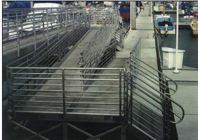
**Figure 17: Up-and-Down Gangway System at Monterey Marina during Operation**
