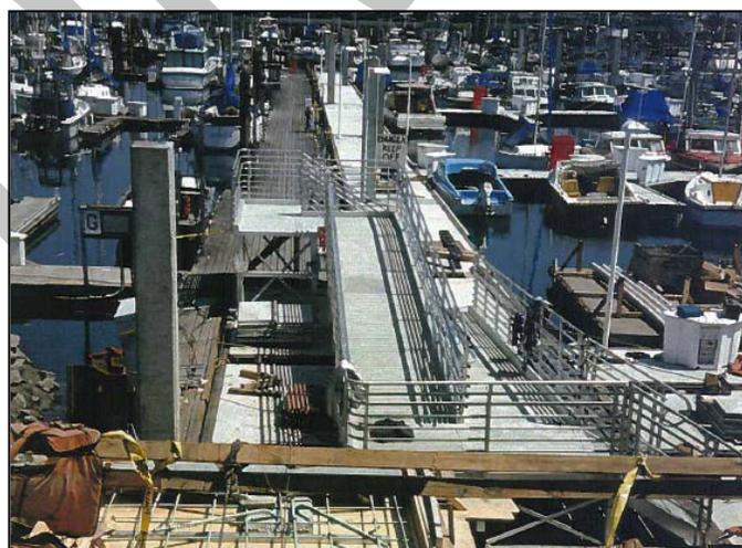
**Figure 16: Up-and-Down Gangway System at Monterey Marina during Construction**
