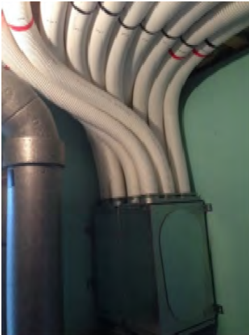
Fig. 4.4 Mixing box (above HRV not shown), with home run ducting (HDPE with smooth interior surface). Image courtesy of NZ Builders.
