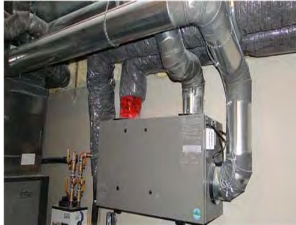
Fig. 4.5 HRV installation with trunk and branch ducting. Insulated ducts are to/from outside.
