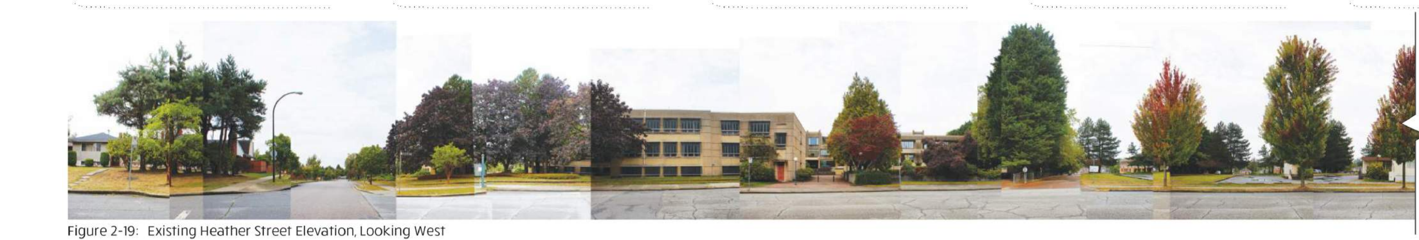
Figure 2-19: Existing Heather Street Elevation, Looking West
