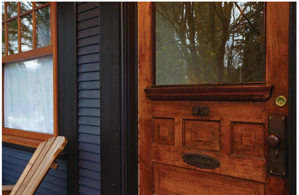
Above: The original windows of this character home had been replaced with aluminum frame windows. In restoring the home, the owner chose to install new, custom wood frame windows that fit with the home's heritage character.
