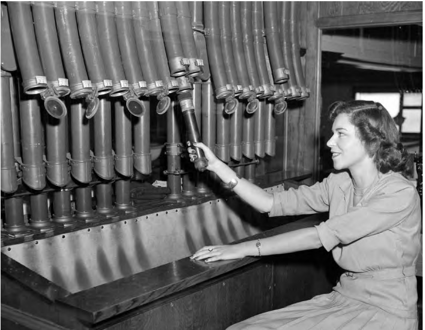
Woman using the pneumatic tube delivery system at the offices of Kelly Douglas Ltd., 1946, CVA 1184-2097
