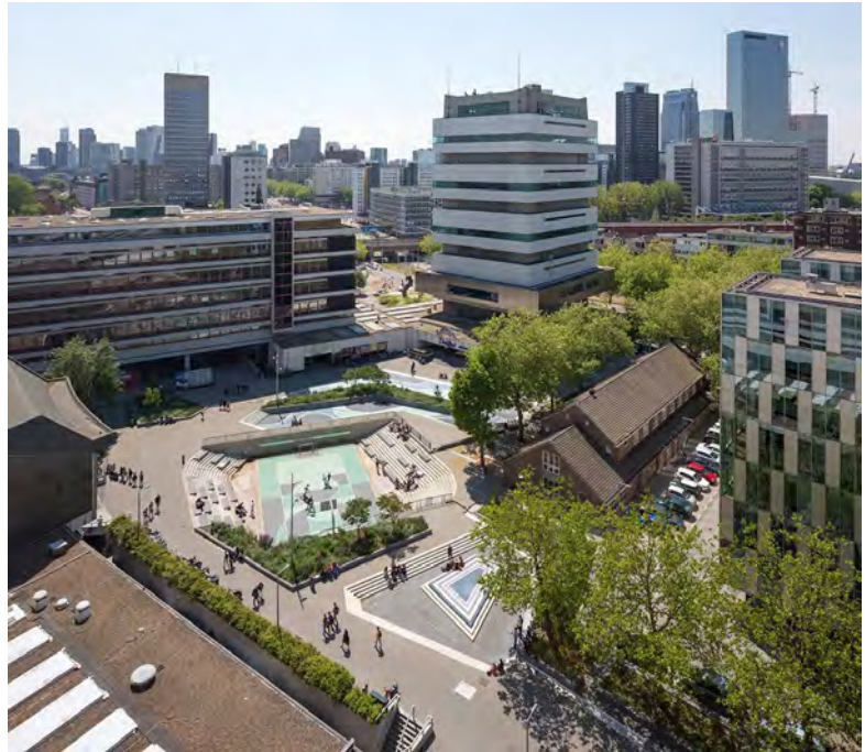
Figure 24: Example of Floodable Public Space in Rotterdam
