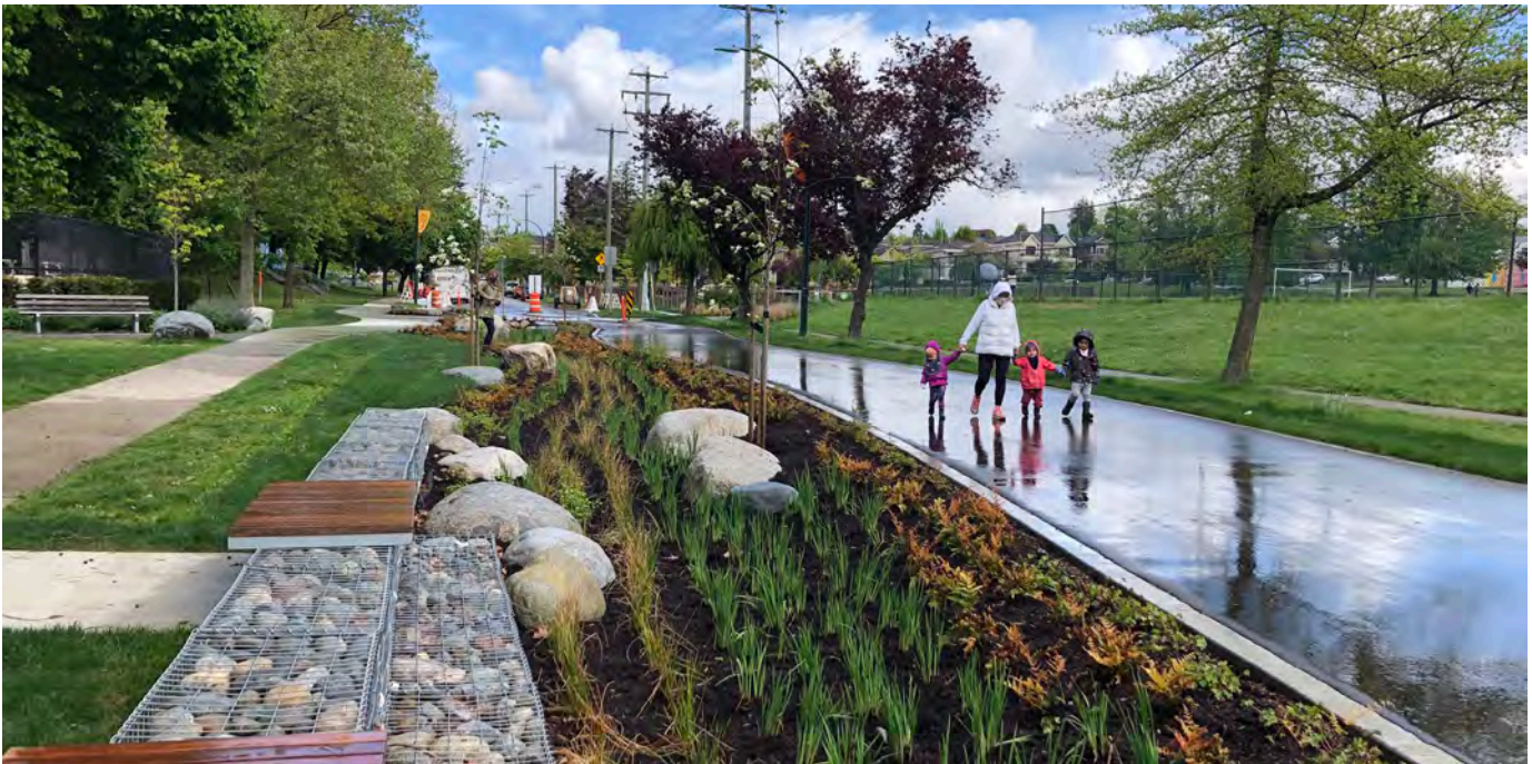
Figure 17: Green Rainwater Infrastructure located on the St George Rainway
