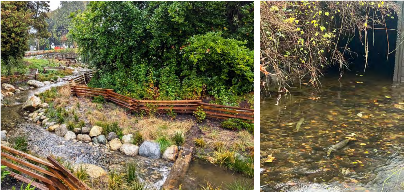
Figure 26: Recent examples of creek daylighting restoration projects at Tatlow Creek (left) and Still Creek (right)
