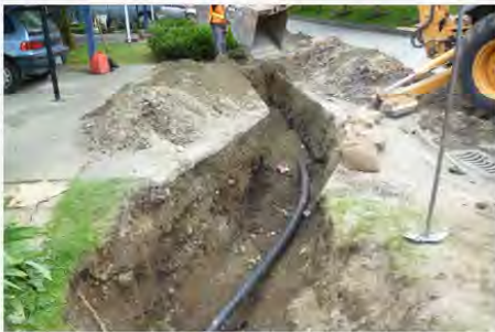
Separating a sewer lateral. (Photo credit: KWL)
