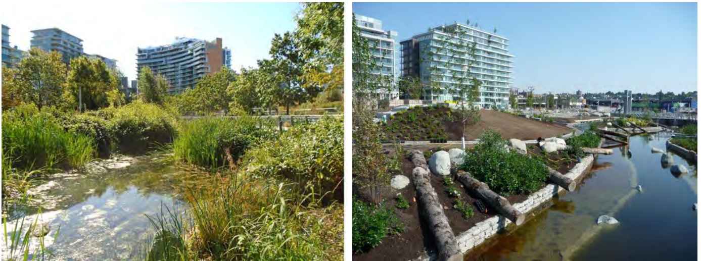
Figure 22: Hinge Park Wetland, a floodable wetland and public space, that includes a constructed wetland with riparian restoration that manages two-thirds of the rainwater that runs off roadways, plazas, and other public spaces in Olympic Village.
