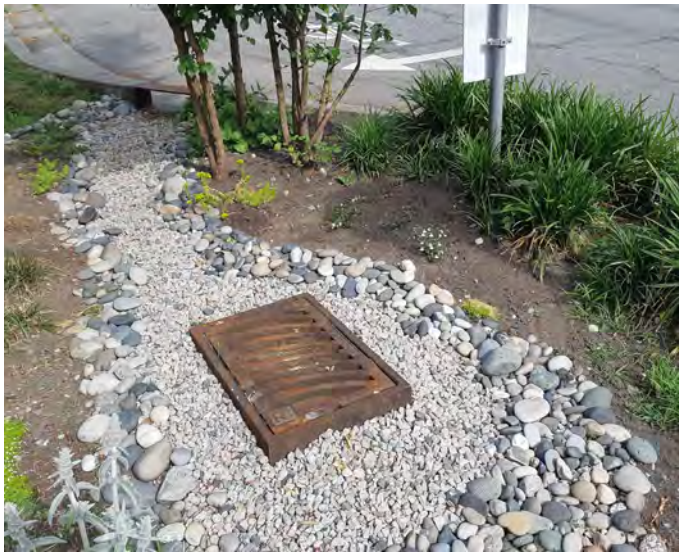
Figure 20: Bioretention bulge (a Green Street feature) at 14 th and Woodland, Vancouver
