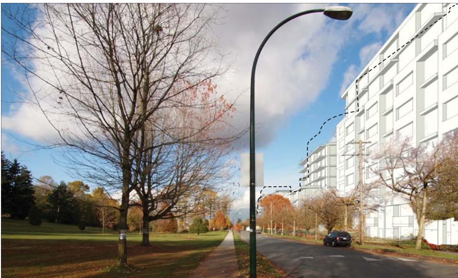
View from Ontario Street near 37 th Avenue looking north
