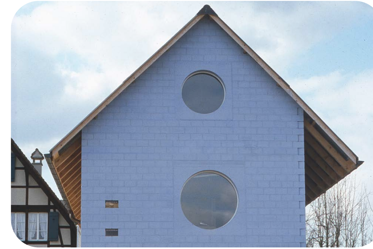
Exteriors: painted concrete block
