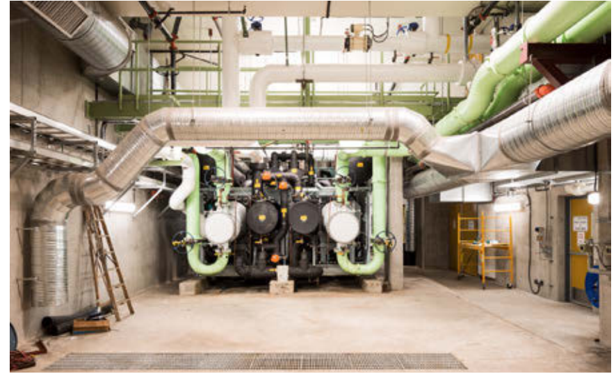
Sewage heat recovery at the Southeast False Creek Energy Centre.
