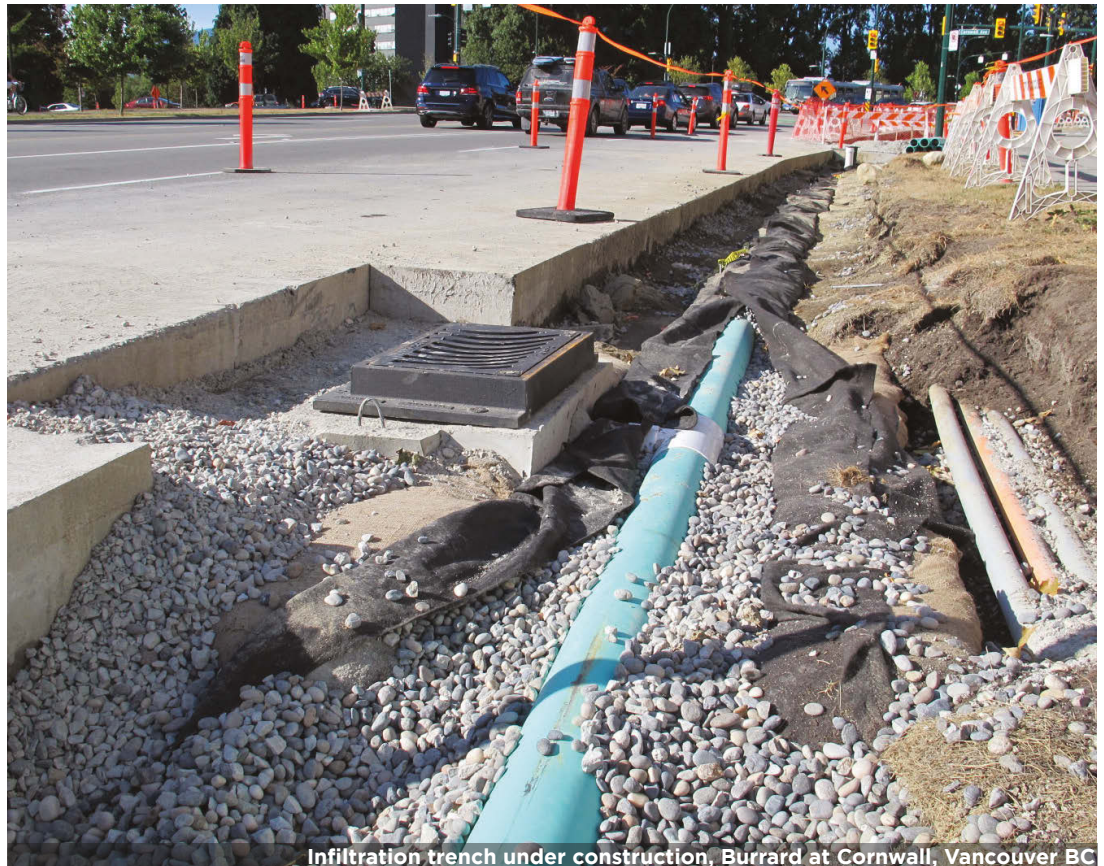
Infiltration trench under construction, Burrard at Cornwall, Vancouver BC
