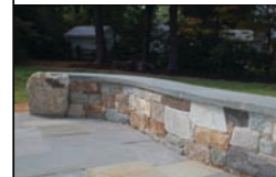
Curved Seating Wall
