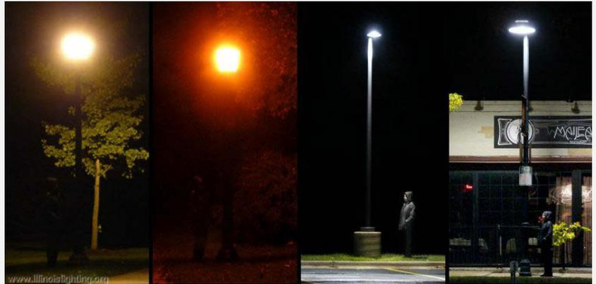
The image above illustrates four different outdoor light fixtures with a person standing beneath each one. The subject is much more visible in the two images on the right, which show **full cut-off** fixtures.
