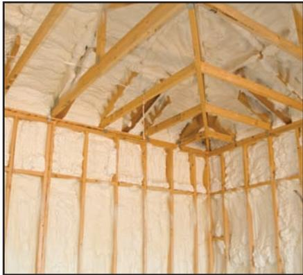
Sprayed foam insulation is used in some higher performance residential buildings. It allows for continuity of insulation as insulation is sprayed when in liquid form, and then expands to fill the cavity – including the smallest cracks. Performance is not as prone to installation errors.
