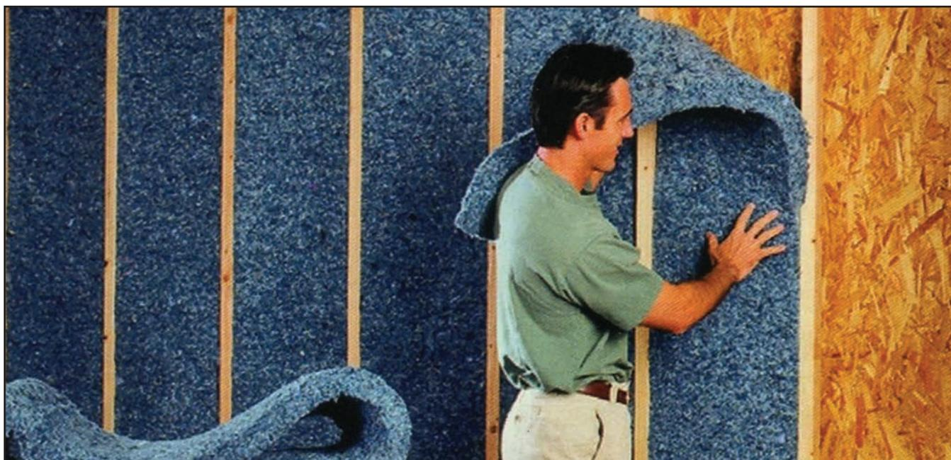
□ **Natural cotton insulation made from recycled or waste denim**
