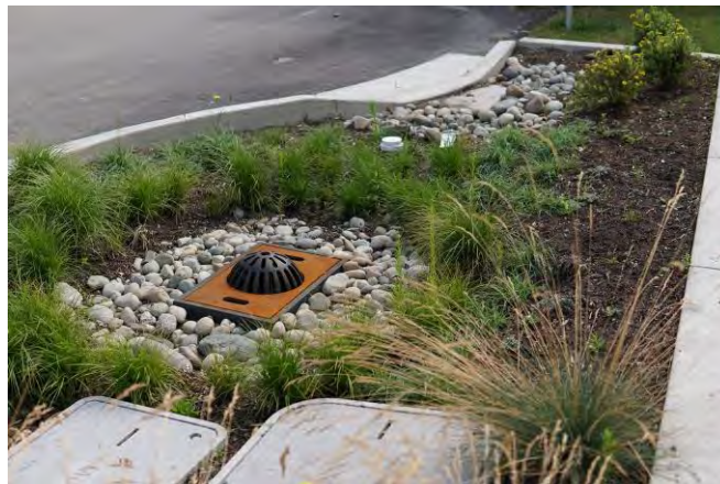
Diagram 4: Curb bulge with green rainwater infrastructure
